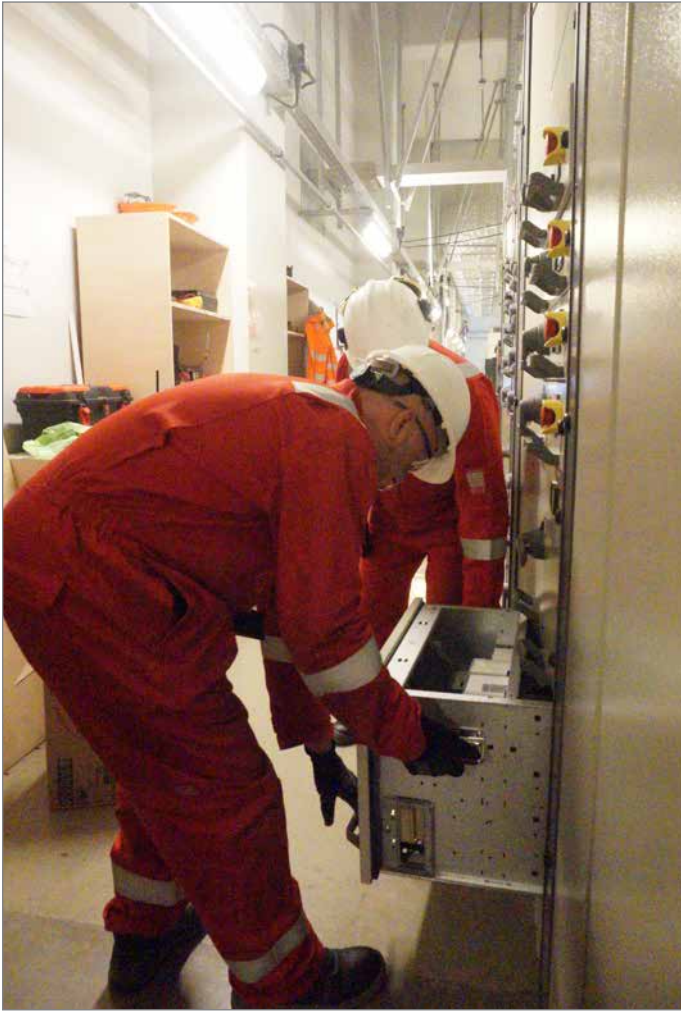
Maintenance of motor control cubicles that power-feed 0.4 kV equipment
