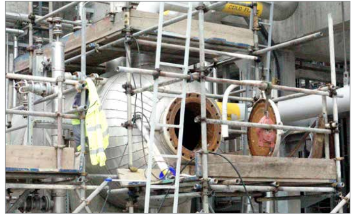
Manhole and blinds of flare drum were dismantled inside, cleaned with a hot water jet, and boxed up with new gaskets
