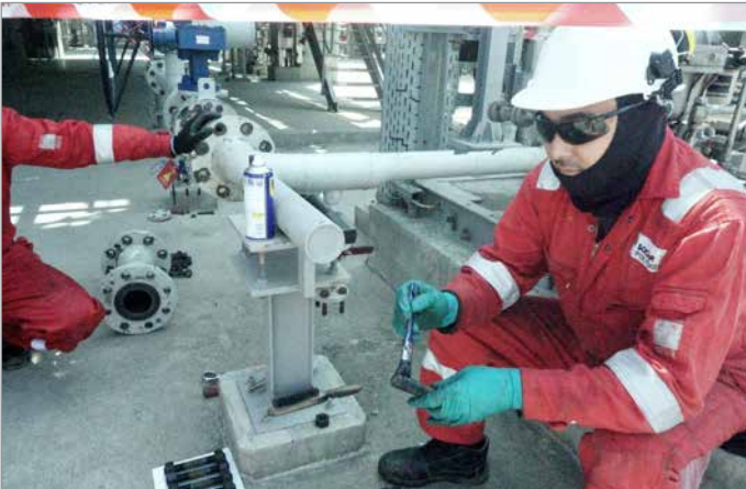
Valve maintenance: fixtures cleaned and lubricated
