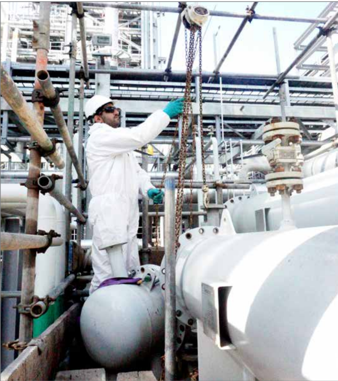
The manhole of the degasser drum was dismantled; the inside of the drum was cleaned, inspected and boxed up
