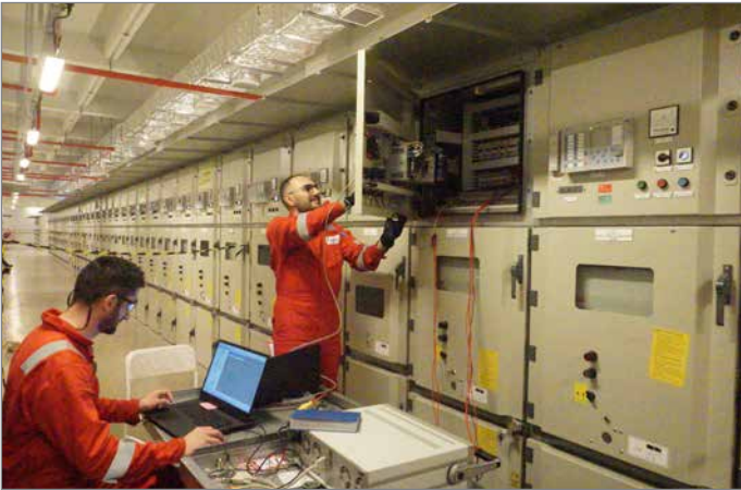
Protection relay and control circuits' testing with Omicron device at the substation
