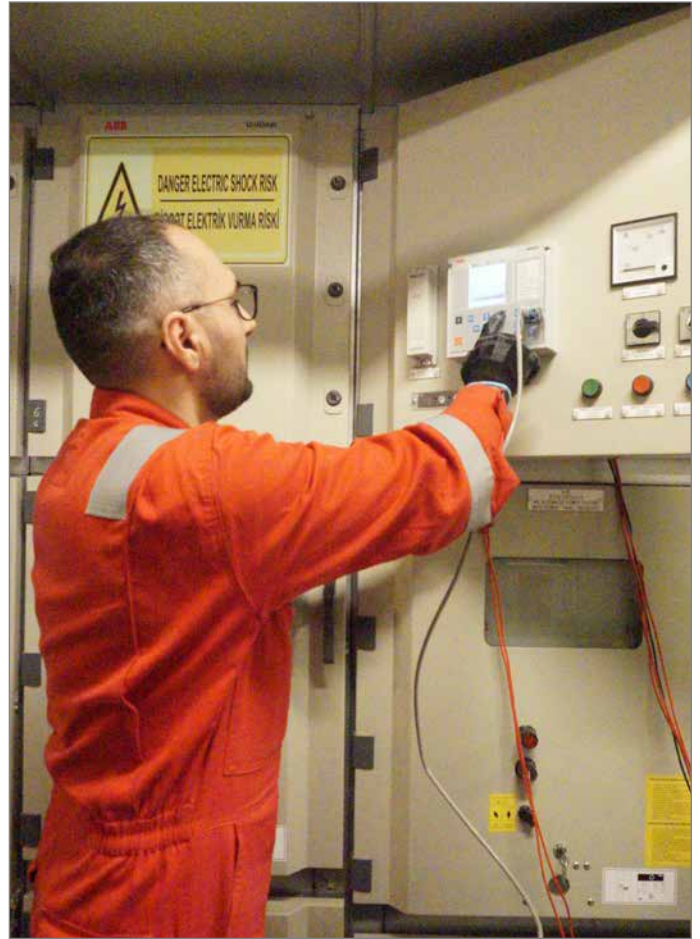
Protection relay and control circuits' testing with Omicron device at the substation
