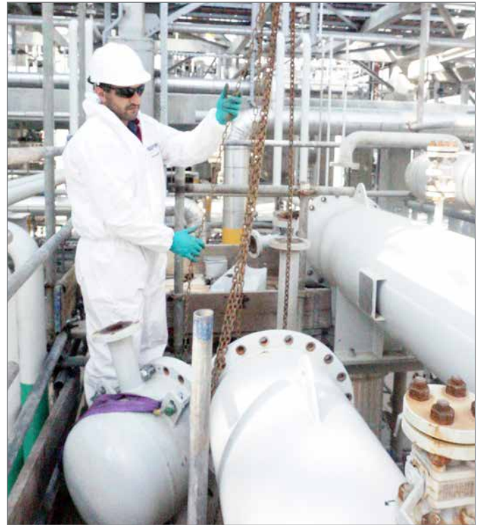
The manhole of the degasser drum was dismantled; the inside of the drum was cleaned, inspected and boxed up
