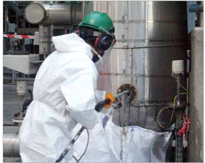
The tube and the shell side of a vertical-type heat exchanger dismantled in the PP polymerization area was cleaned and boxed up
