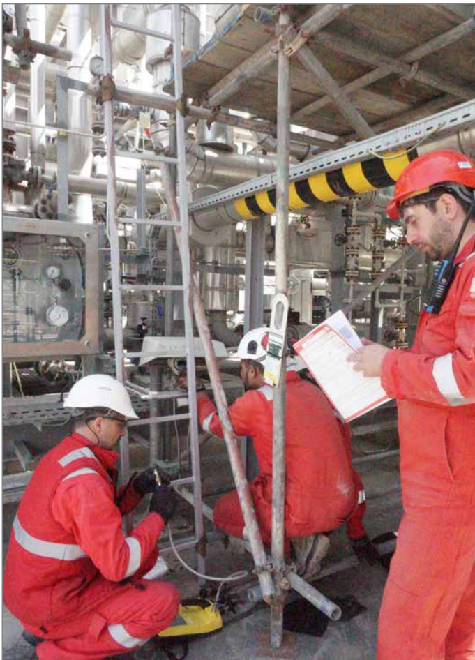
Recalibration of a level transmitter
