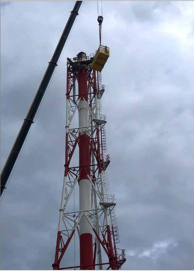
Installation of a retractable system for aircraft warning lights on the flare
