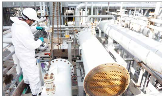
A mechanical technician dismantled, cleaned, and boxed up of a horizontal-type shell-and-tube heat exchanger in the HDPE polymerization area.
