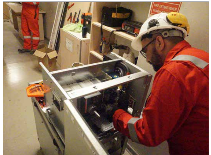
Protection relay and control circuits' testing with Omicron device at the substation
