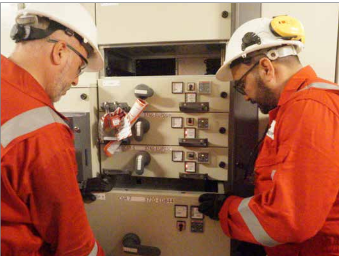
Protection relay and control circuits' testing with Omicron device at the substation
