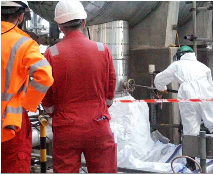
The tube and the shell side of a vertical-type heat exchanger dismantled in the PP polymerization area was cleaned and boxed up
