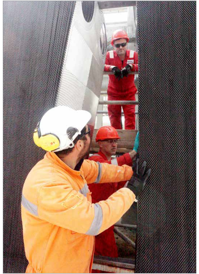
Gasket strips placed back onto heat exchanger plates
