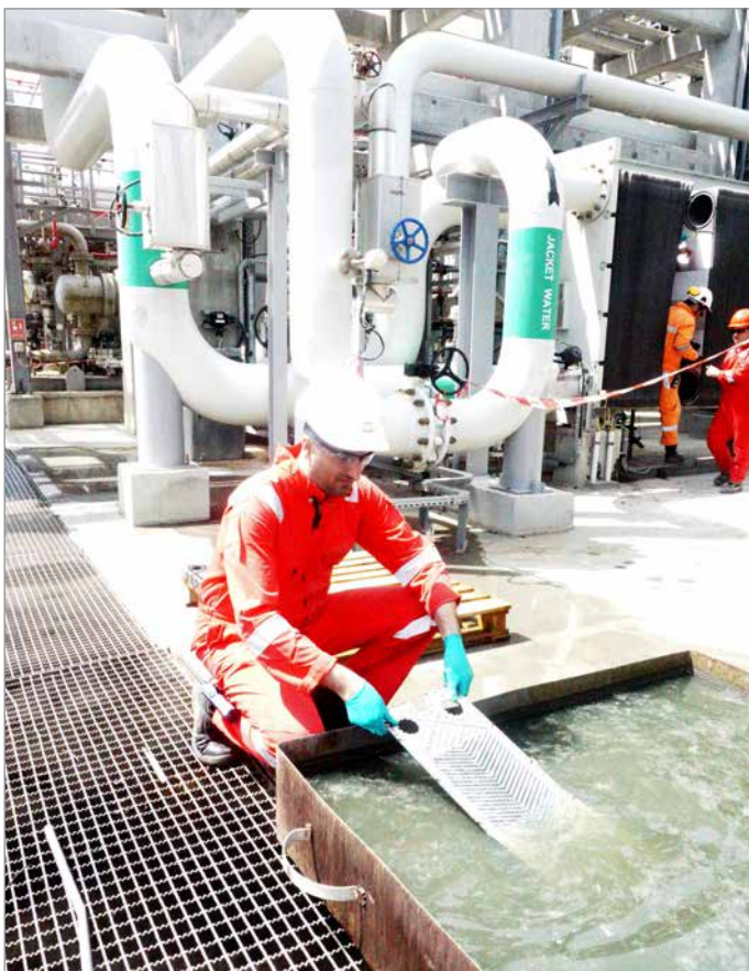
Heat exchanger plates washed in cleansing solution
