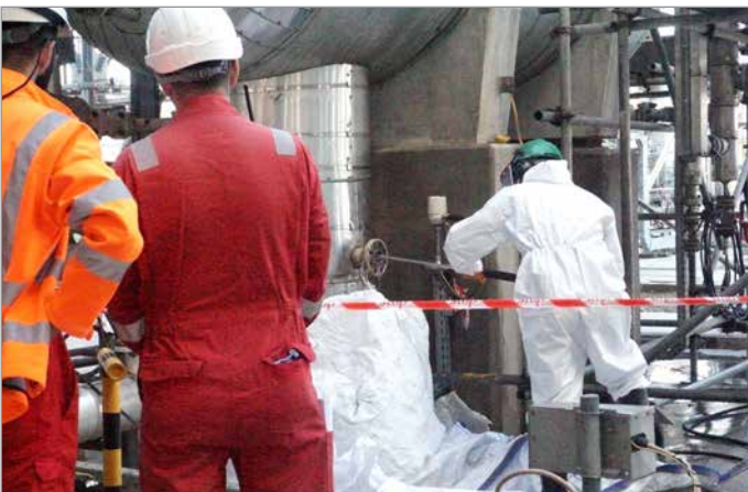
D-1912 flare drum cleaning with hot water jetting
