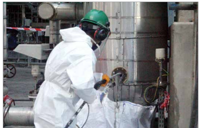
Manhole and blinds of flare drum were dismantled inside, cleaned with a hot water jet, and boxed up with new gaskets
