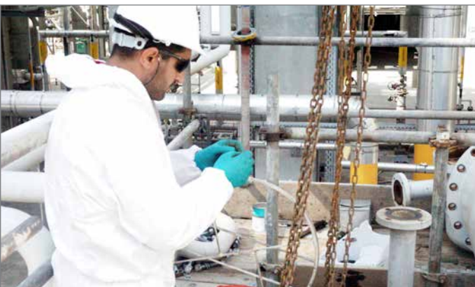
A mechanical technician dismantled, cleaned, and boxed up of a horizontal-type shell-and-tube heat exchanger in the HDPE polymerization area.
