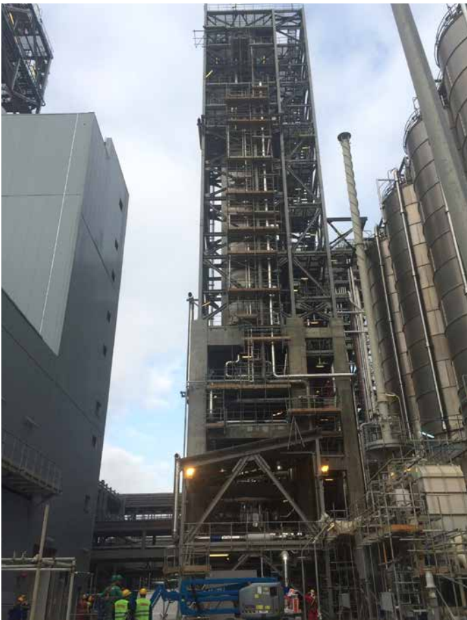
HDPE: Organoleptic Structure and Effluent Treatment. Piping installation ongoing
