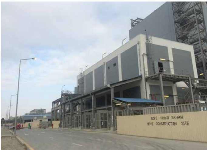
HDPE: Electrical Substation. Cabling and termination completed
