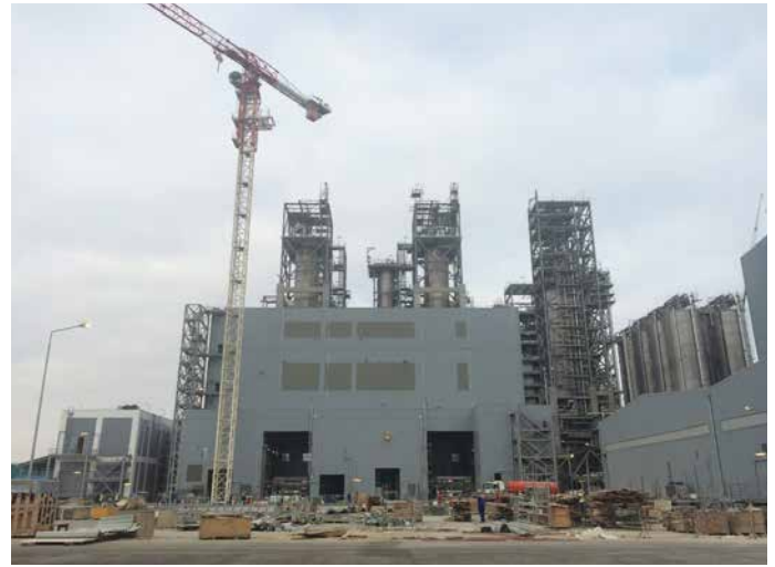
HDPE: Extrusion Structure. Piping insulation completed. Doors installation almost completed
