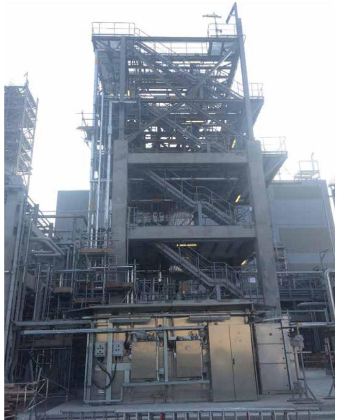
HDPE: Low Pressure Solvent Recovery. Piping insulation and painting works ongoing
