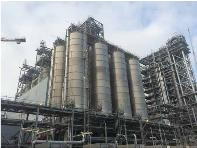
HDPE: Blending Silos. Piping insulation ongoing
