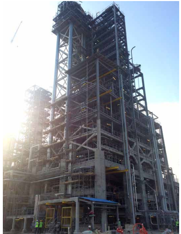
HDPE: Polymerization. Cable tray cover installation and piping insulation works ongoing
