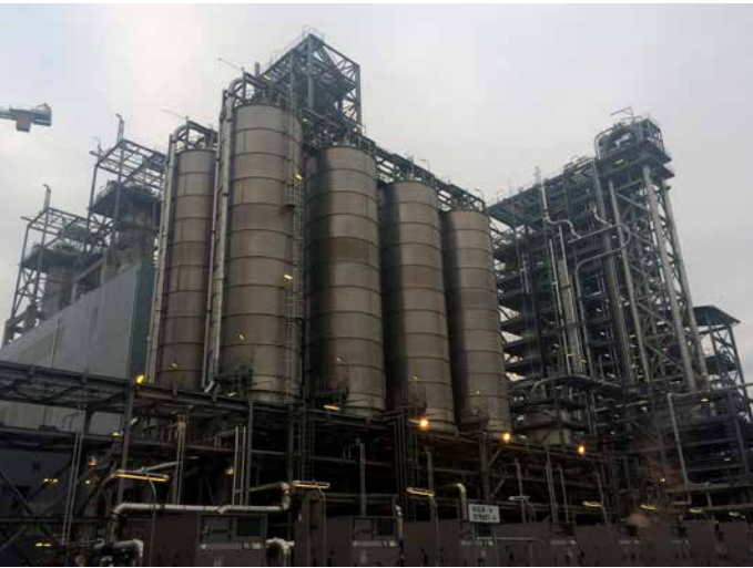
HDPE: Blending Silos. Punch clearance ongoing
