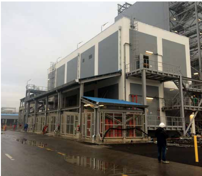
HDPE: Electrical Substation. Punch clearance ongoing
