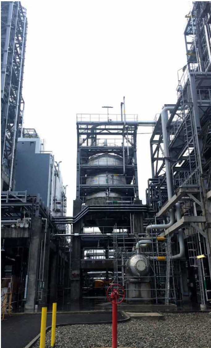
HDPE: Reactor Dump tank. Punch clearance in progress
