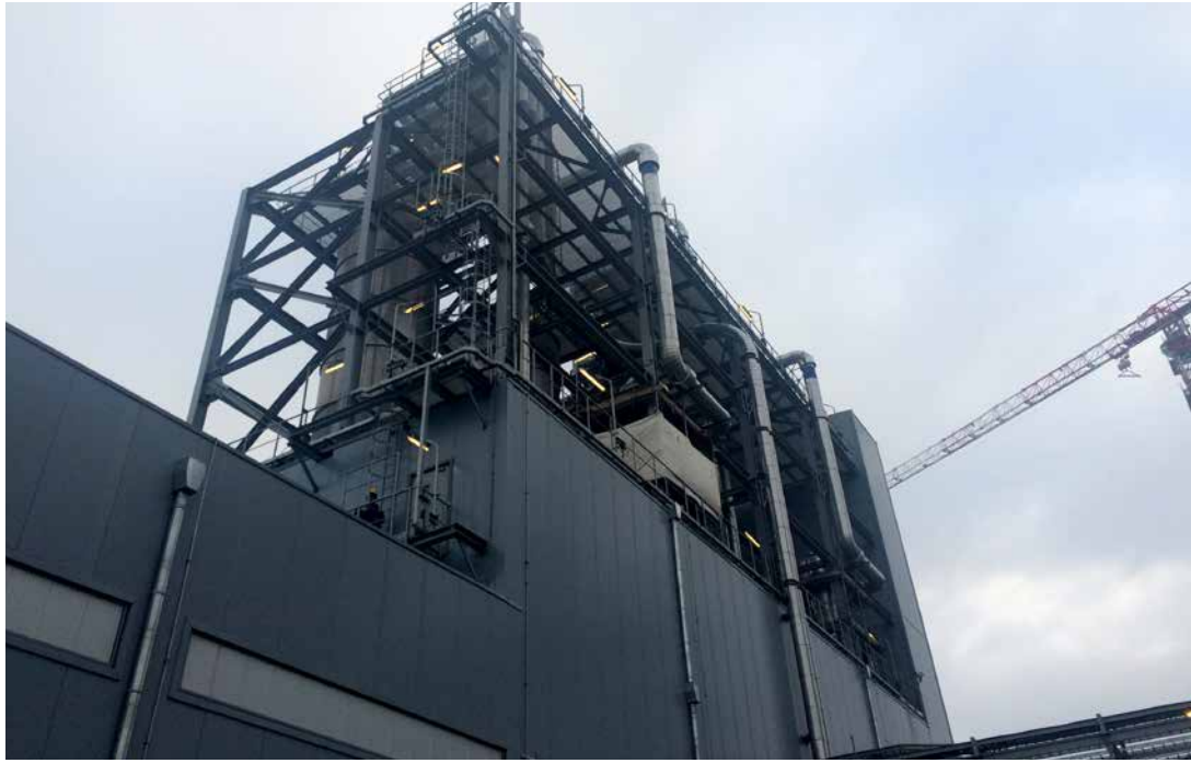
HDPE: Bagging & Packing. Punch clearance in progress
