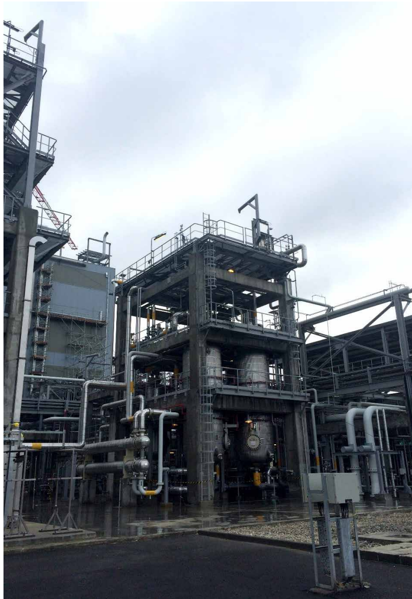
HDPE: Ethylene Treatment. Punch clearance in progress
