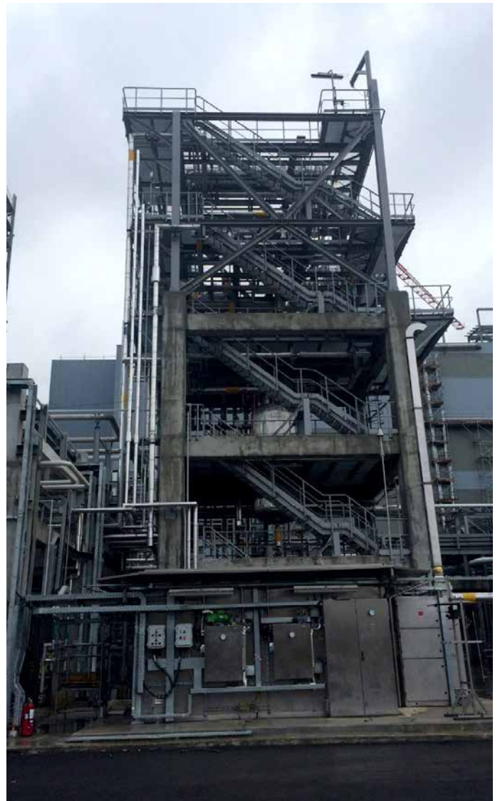
HDPE: Low Pressure Solvent Recovery. Punch clearance in progress
