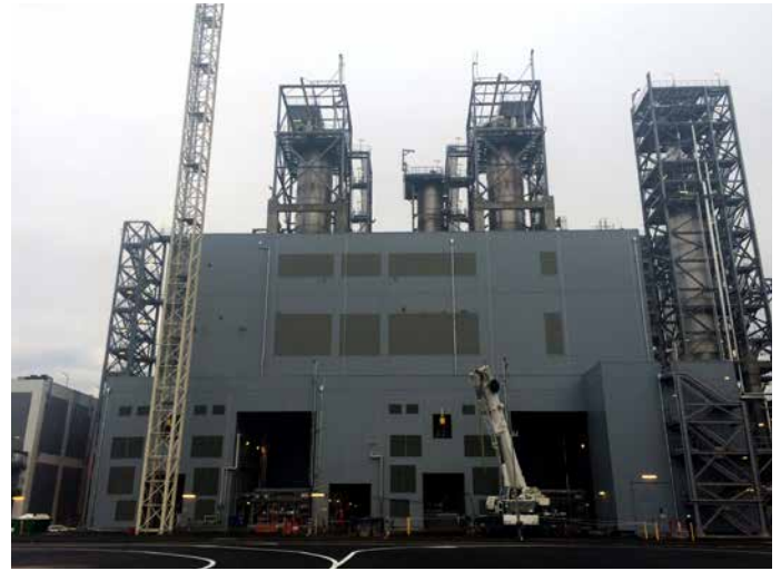
HDPE: Extrusion Structure. Punch clearance in progress
