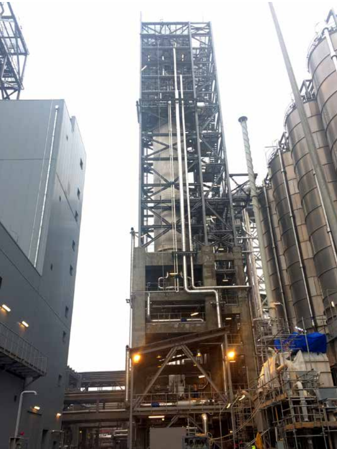
HDPE: Organoleptic Structure and Effluent Treatment. Punch clearance ongoing
