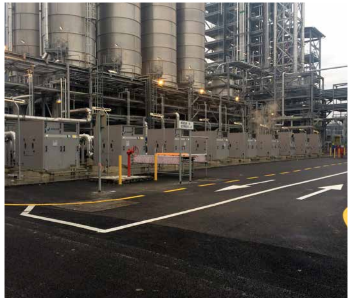
HDPE: Pellet blower package space for logistic conveying. Punch clearance in progress
