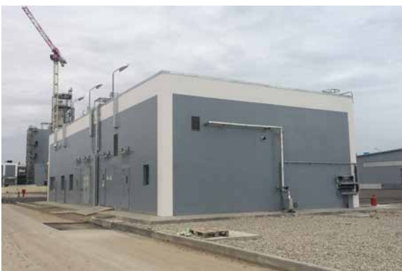
PP/U&O: Administration building. Punch List closing in progress
