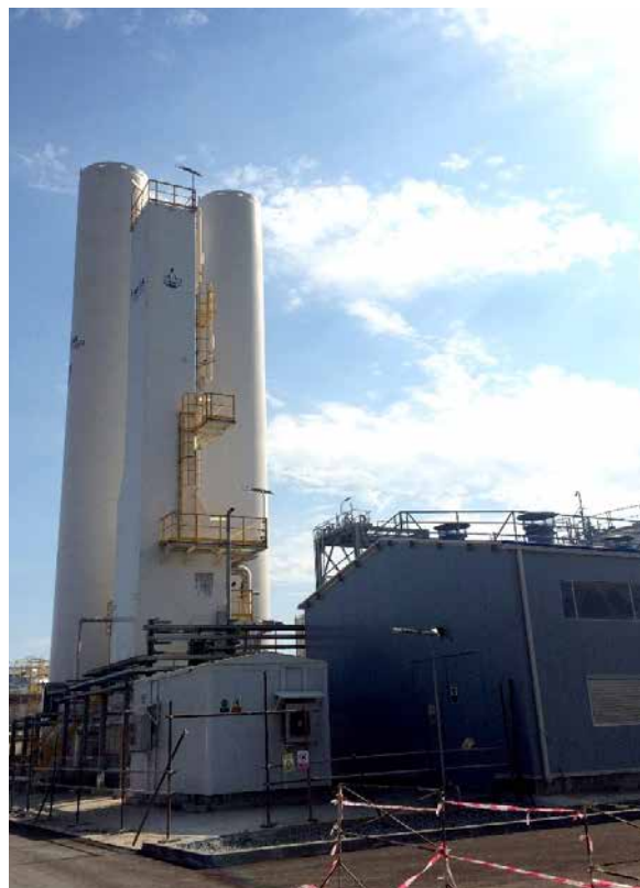
Nitrogen package. Construction works completed
