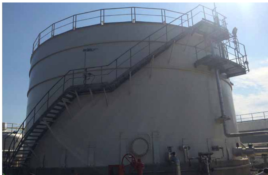
PP/U&O: Raw Water Storage Tank. Punch List closing in progress
