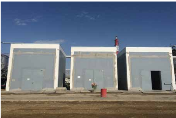
PP/U&O: Valve house. Punch List closing in progress
