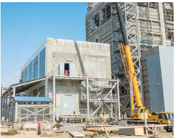
HDPE: Polymerization. Reactor Circulation Pumps and the Bottom elbow part of Loop Reactors erected. Structural & piping erection works for Remote Operator Monitors ongoing
