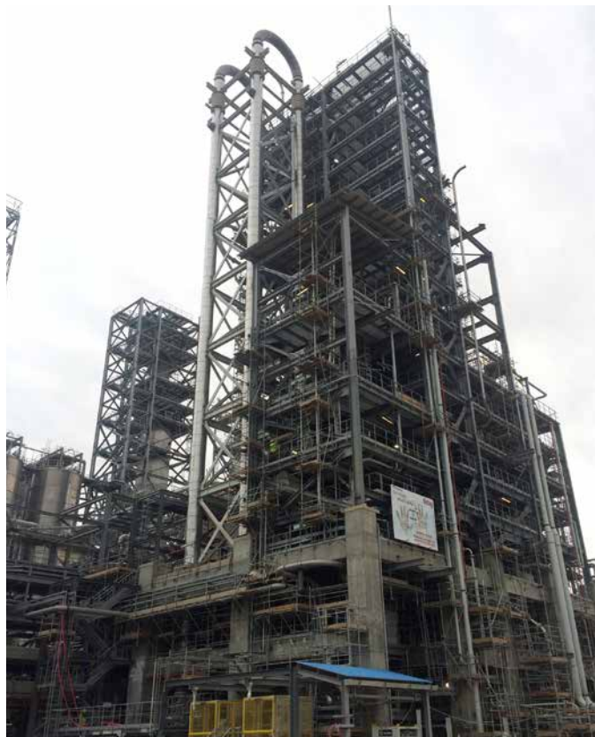
HDPE: Polymerization. Reactor Circulation Pumps and the Bottom elbow part of Loop Reactors erected. Structural & piping erection works for Remote Operator Monitors ongoing
