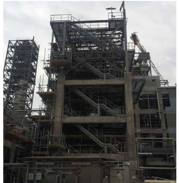
HDPE: Low Pressure Solvent Recovery. Equipment Insulation completed on E-1414 and D-1425. Piping insulation and painting ongoing
