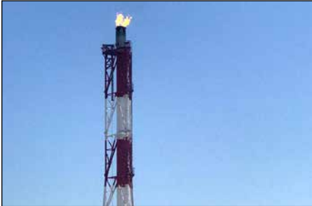
Hydrocarbon feedstock introduced to the PP plant p.16
