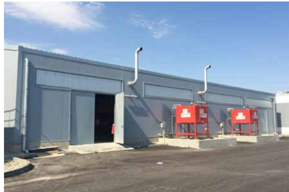
PP/U&O: Fire water Retention Basins and Pump House. Commissioning in progress
