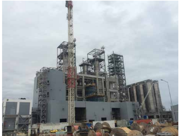
HDPE: Extrusion Structure. Secondary steel, hand rails & grating works ongoing at the top of the silos. Piping erection and painting in progress
