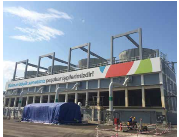
PP/U&O: Cooling Tower. Punch List closing in progress
