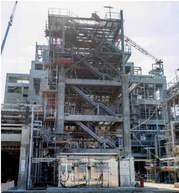
HDPE: Low Pressure Solvent Recovery. Equipment Insulation completed on E-1414 and D-1425. Piping insulation and painting ongoing
