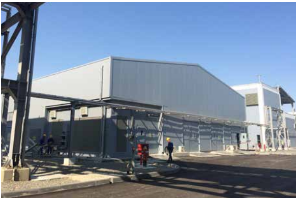
PP/U&O: Chemical & Additives Storage Building. Punch List closing in progress
