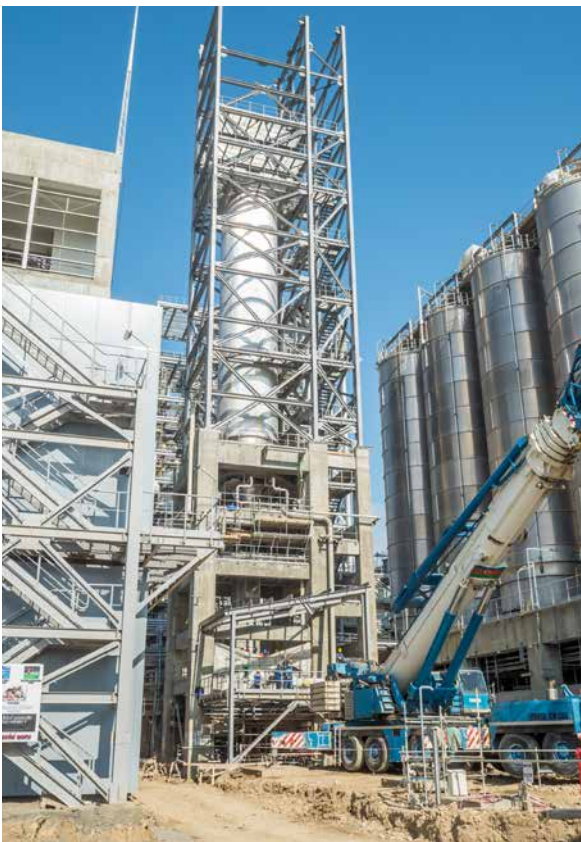
HDPE: Organoleptic Structure and Effluent Treatment. Secondary steel and grating works ongoing on final level. Instrument installation and cooling water lines' erection in progress
