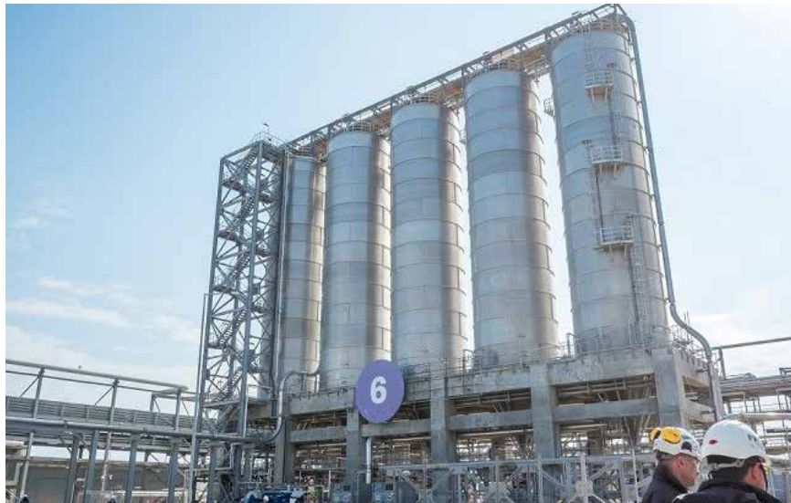
PP/U&O: Homogenization / Blender Silos. Punch List closing in progress
