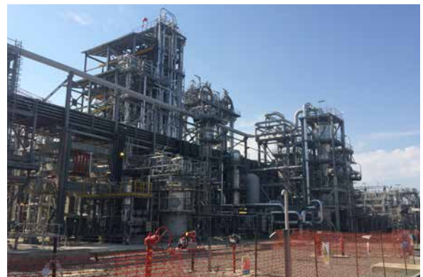
PP/U&O: PP-Wet section / Polymerization. Punch List closing in progress
