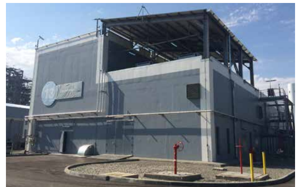
PP/U&O: Laboratory. Punch List closing in progress
