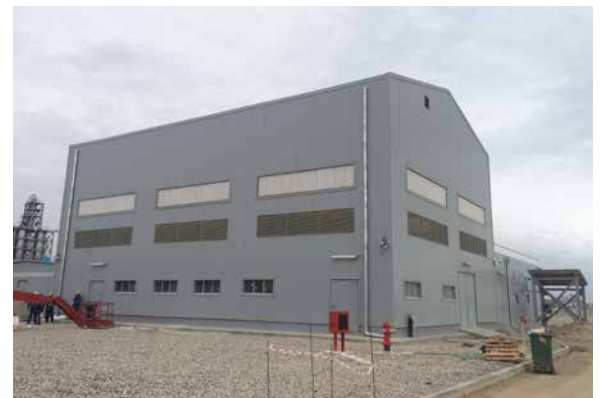
PP/U&O: Workshop. Punch List closing in progress
