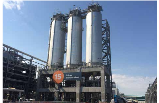
PP/U&O: PP Dry section / Powder Silos. Punch List closing in progress
