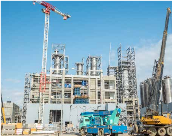
HDPE: Extrusion Structure. Secondary steel, hand rails & grating works ongoing at the top of the silos. Piping erection and painting in progress
