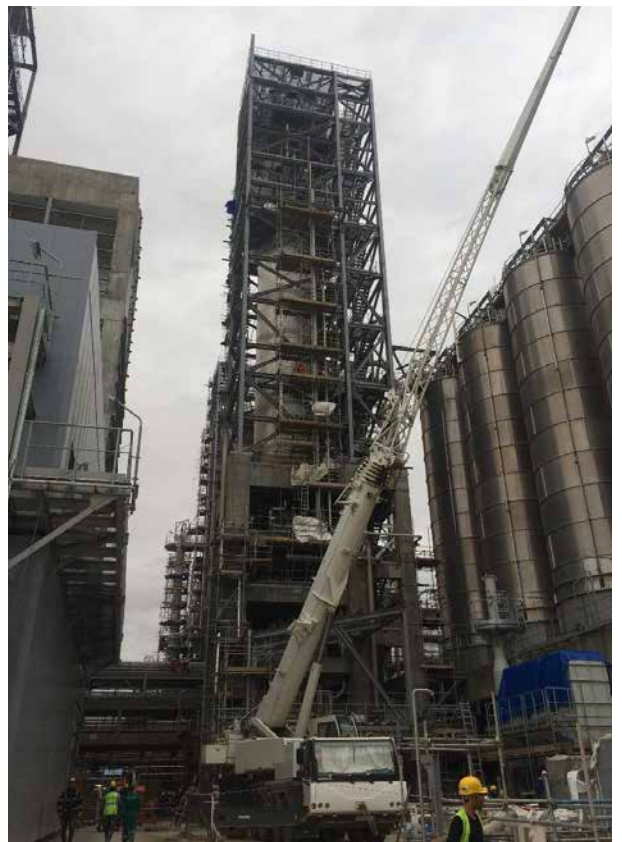
HDPE: Organoleptic Structure and Effluent Treatment. Secondary steel and grating works ongoing on final level. Instrument installation and cooling water lines' erection in progress
