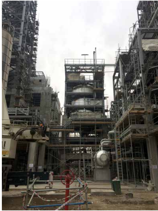
HDPE: Reactor Dump tank. Electrical works in progress
