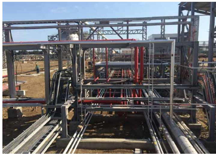
PP/U&O: Interconnecting Pipe Racks. ICPR 800, 801, 802, 803, 804, 807, 809, 810, 819 Punch List closing in progress
