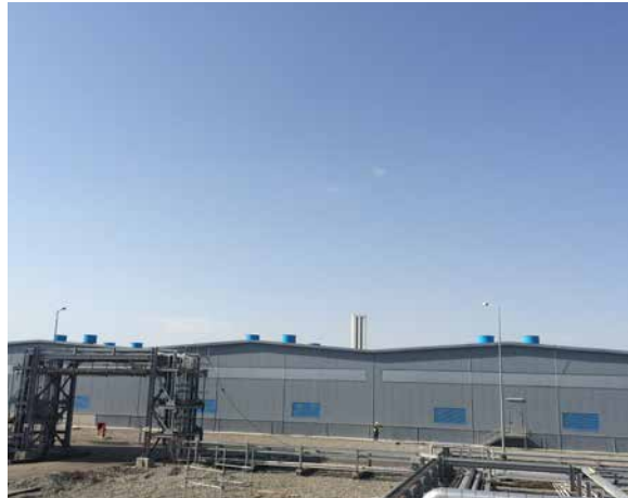
Warehouse. Joint sealing works in progress
