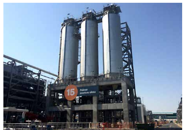
PP/U&O: PP Dry section / Powder Silos. Punch List closing in progress
