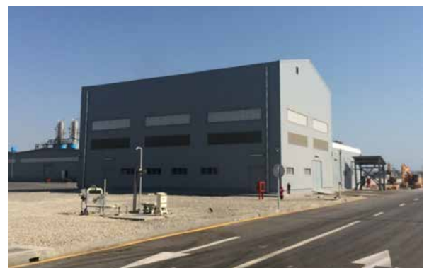
PP/U&O: Workshop. Punch List closing in progress
