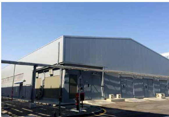
PP/U&O: Chemical & Additives Storage Building. Punch List closing in progress
