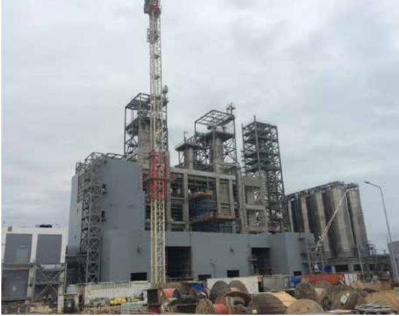
HDPE: Extrusion Structure. Roof insulation, sandwich panels and gypsum board installation works are ongoing. Piping erection and painting in progress
