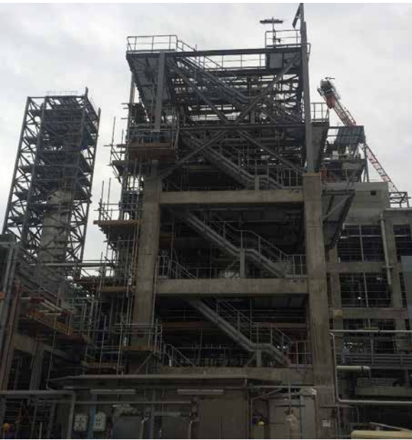
HDPE: Low Pressure Solvent Recovery. Hydrotest ongoing. Piping insulation and painting works ongoing
