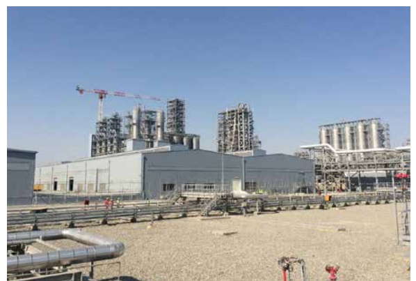
PP/U&O: Bagging & Packing Building. Punch List closing in progress
