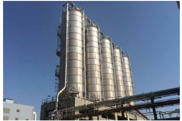
PP/U&O: Homogenization / Blender Silos. Punch List closing in progress
