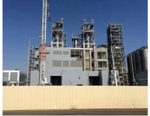
HDPE: Extrusion Structure. Roof insulation, sandwich panels and gypsum board installation works are ongoing. Piping erection and painting in progress
