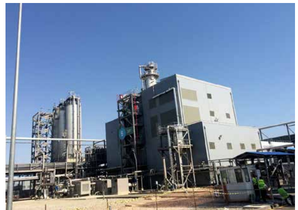
PP/U&O: PP Dry Section / Extrusion building. Punch List closing in progress
