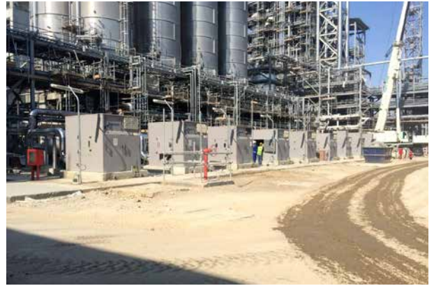
HDPE: Pellet blower package space for logistic conveying. Piping works ongoing
