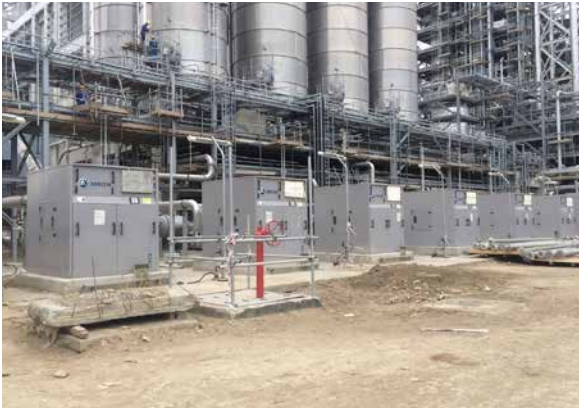
HDPE: Pellet blower package space for logistic conveying. Piping works ongoing
