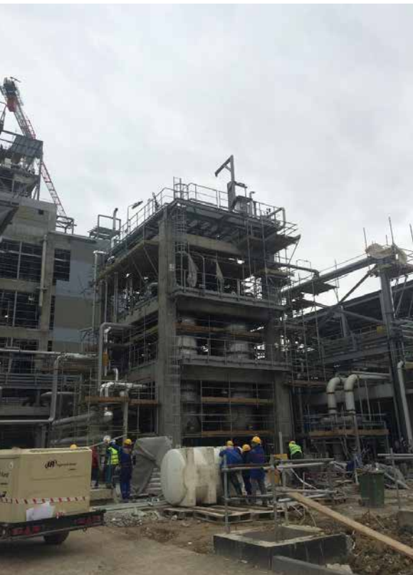
HDPE: Ethylene Treatment. Piping insulation and painting works ongoing
