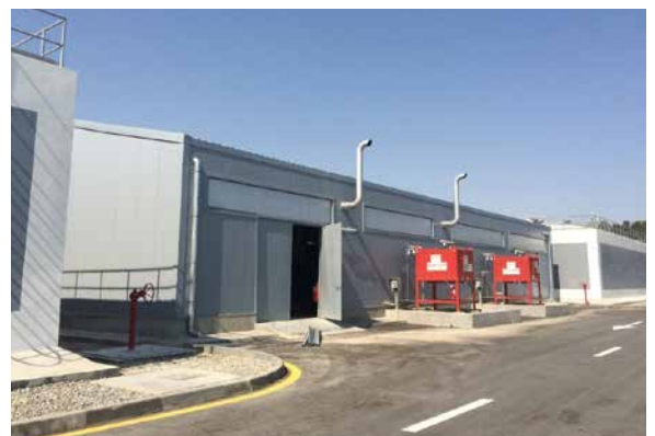
PP/U&O: Fire water Retention Basins and Pump House. All works completed
