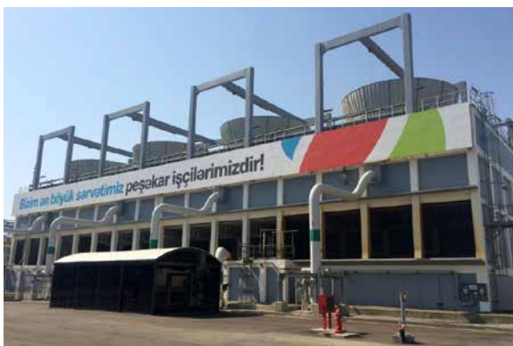
PP/U&O: Cooling Tower. Punch List closing in progress
