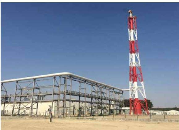
PP/U&O: Flare Stack. Punch List closing in progress
