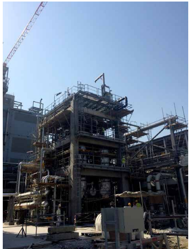
HDPE: Ethylene Treatment. Piping insulation and painting works ongoing
