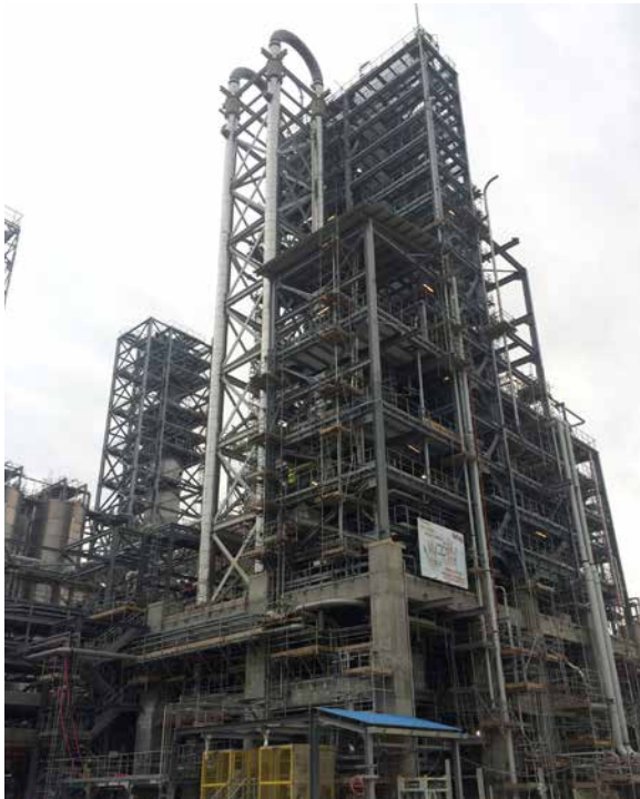
HDPE: Polymerization. Structural & piping works for Remote Operator Monitors are ongoing. Equipment cable connection ongoing
