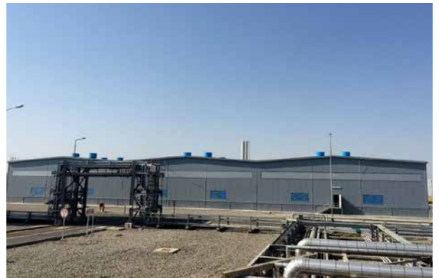
Warehouse. Joint sealing works completed. Painting works in progress
