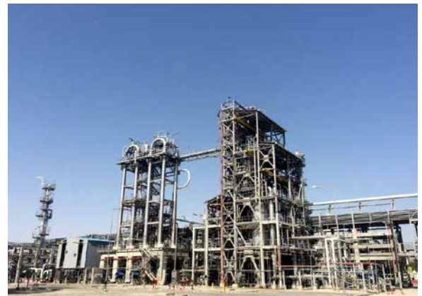
PP/U&O: PP-Wet section / Polymerization. Punch List closing in progress
