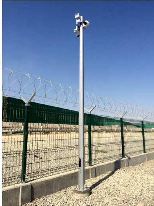
Permanent PS System. Cable pulling in progress
