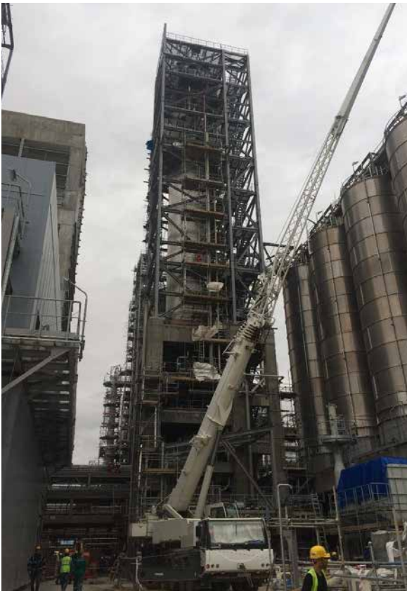
HDPE: Organoleptic Structure and Effluent Treatment. Instrument installation and cooling water lines erection ongoing
