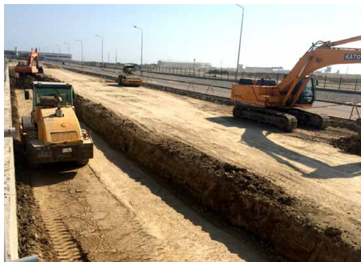
Roads. Excavation and compaction works in progress
