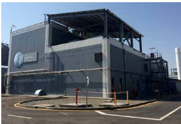
PP/U&O: Laboratory. Punch List closing in progress
