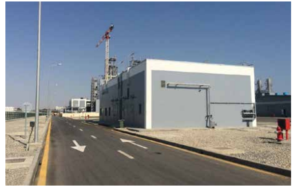
PP/U&O: Administration building. Punch List closing in progress
