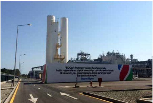
Nitrogen package. Works completed
