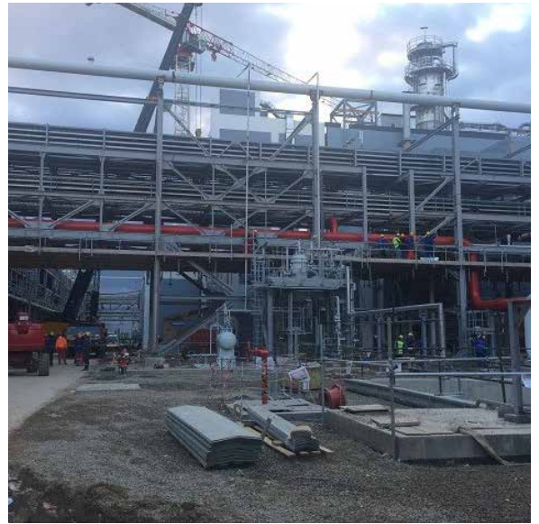
PP/U&O: Interconnecting Pipe Racks. Pipe testing in progress. Cable pulling ongoing
