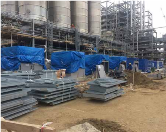
HDPE: Pellet blower package space for logistic conveying. Pipe erection in progress
