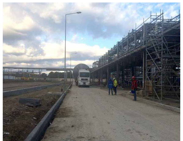
Roads. Internal roads' construction ongoing. Laying of the first asphalt layer ongoing. Area lighting works in progress
