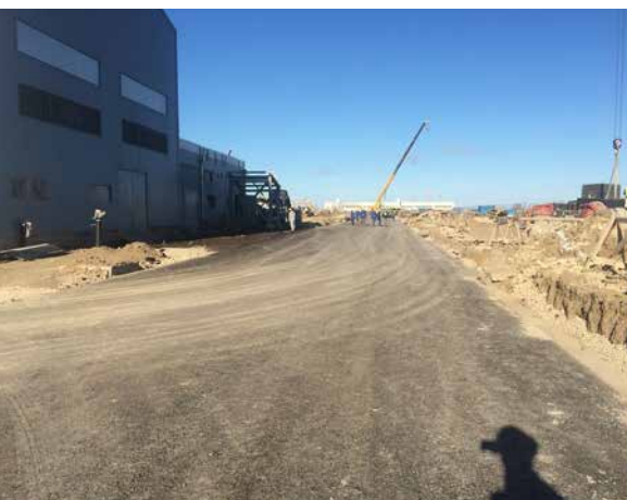
Roads. Internal roads' construction ongoing. Laying of the first asphalt layer ongoing. Area lighting works in progress
