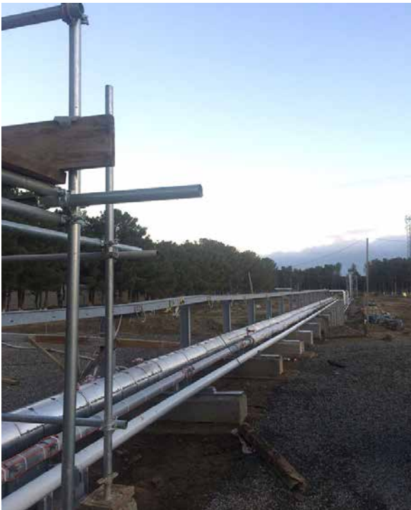
PP/U&O: Pipe Sleepers. Pipe erection and cable tray installation ongoing
