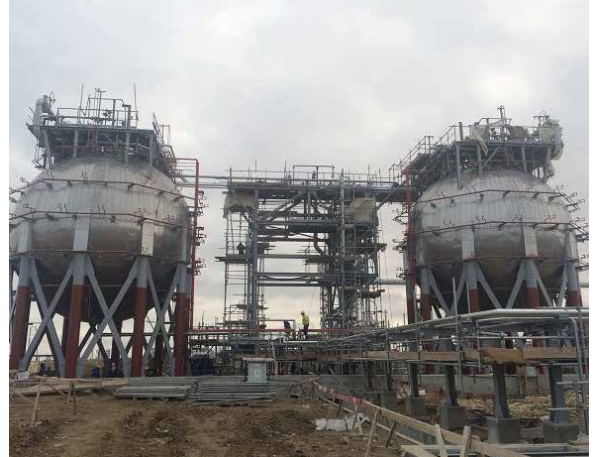
PP/U&O: Isobutane Sphere. Sprinkler system installation completed
