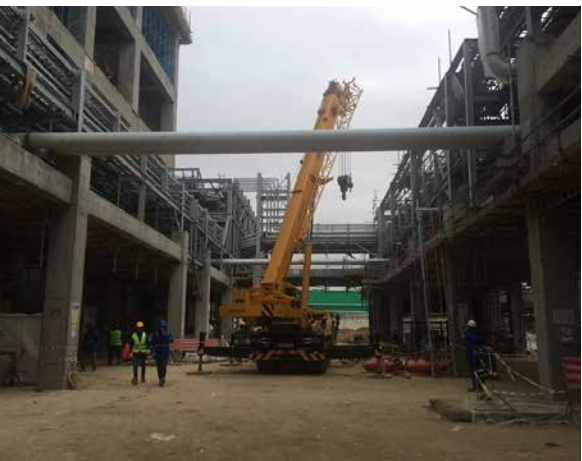
HDPE: Polymerization Pipe Rack. Pipe support installation ongoing. Cable tray installation ongoing. Cable pulling in progress
