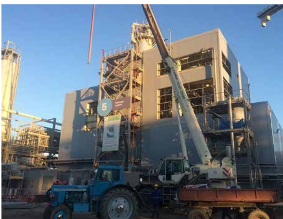
PP/U&O: PP Dry Section / Extrusion building. Most piping tests completed. Lighting System installed and powered up. Lift erection in progress
