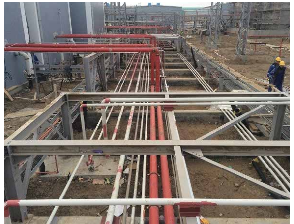
PP/U&O: Pipe Sleepers. Pipe erection and cable tray installation ongoing
