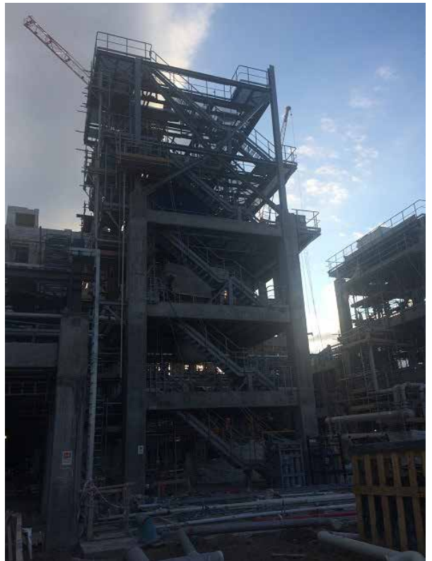
HDPE: Low Pressure Solvent Recovery. SS erection in progress
