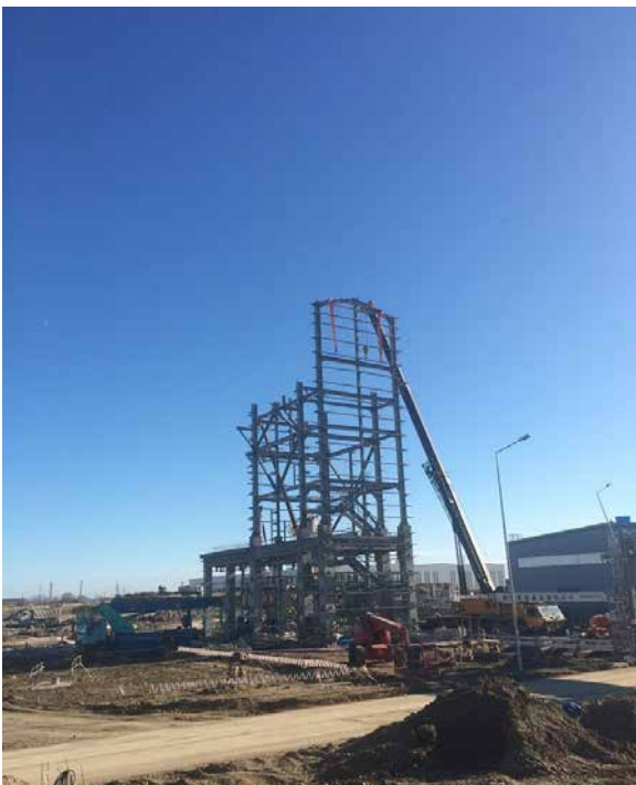
HDPE: Catalyst Activation. SS erection in progress
