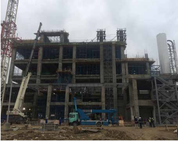
HDPE: Extrusion Structure. RCC works completed. SS and piping erection in progress
