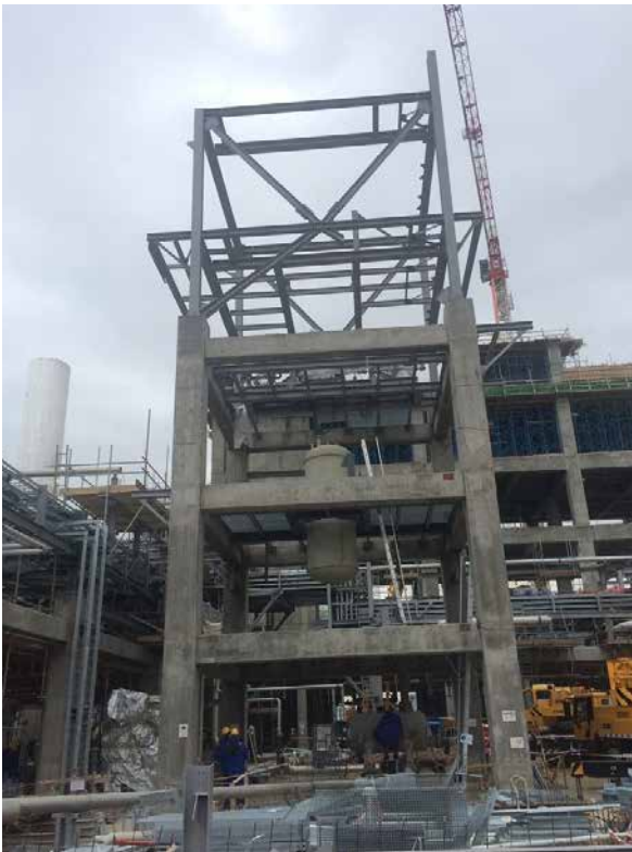
HDPE: Low Pressure Solvent Recovery. SS erection in progress
