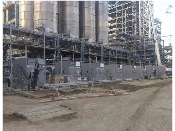
HDPE: Pellet blower package space for logistic conveying. Pipe erection in progress
