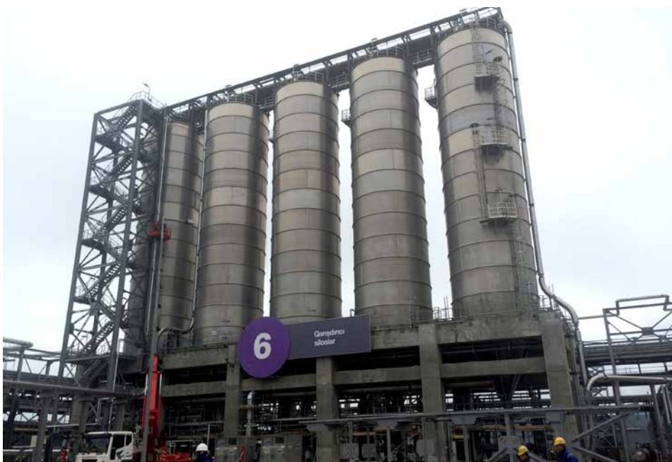
PP/U&O: Homogenization / Blender Silos. Pre-commissioning activities in progress
