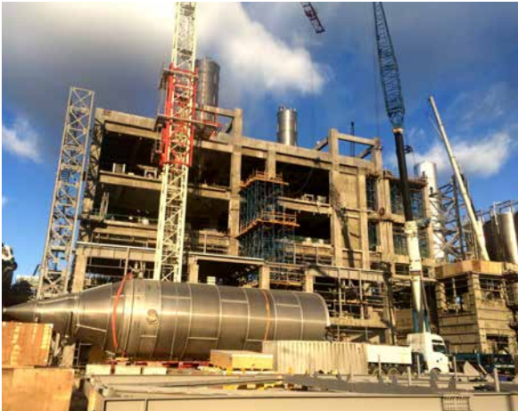
HDPE: Extrusion Structure. RCC works completed. SS and piping erection in progress. Junction box and sandwich panel installation in progress
