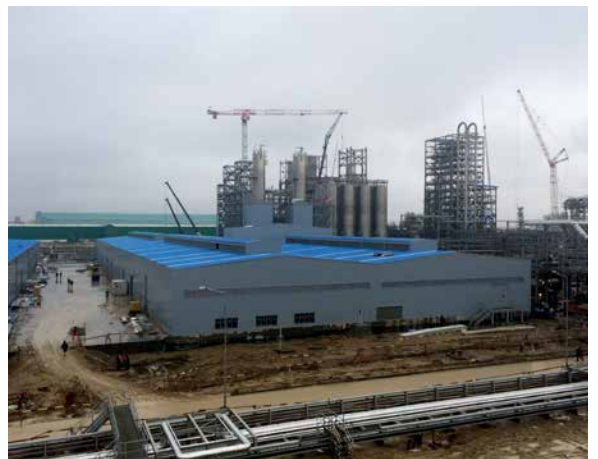
PP/U&O: Bagging & Packing Building. Wall and roof sheeting installation in progress
