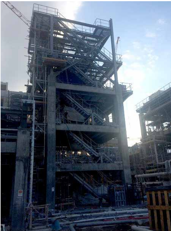
HDPE: Low Pressure Solvent Recovery. Instrument installation and cabling complete
