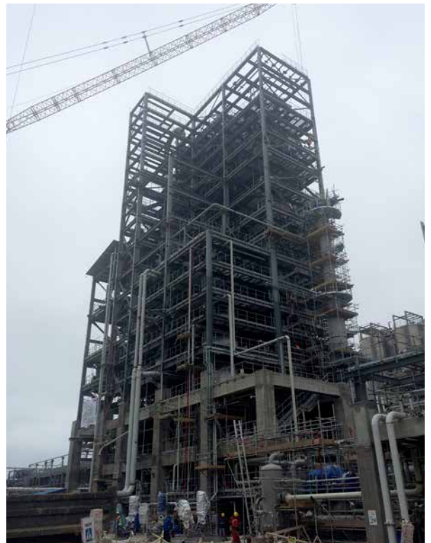
HDPE: Polymerization. Equipment erected. Piping & Support erection ongoing. SS, junction box, lighting etc. installation in progress
