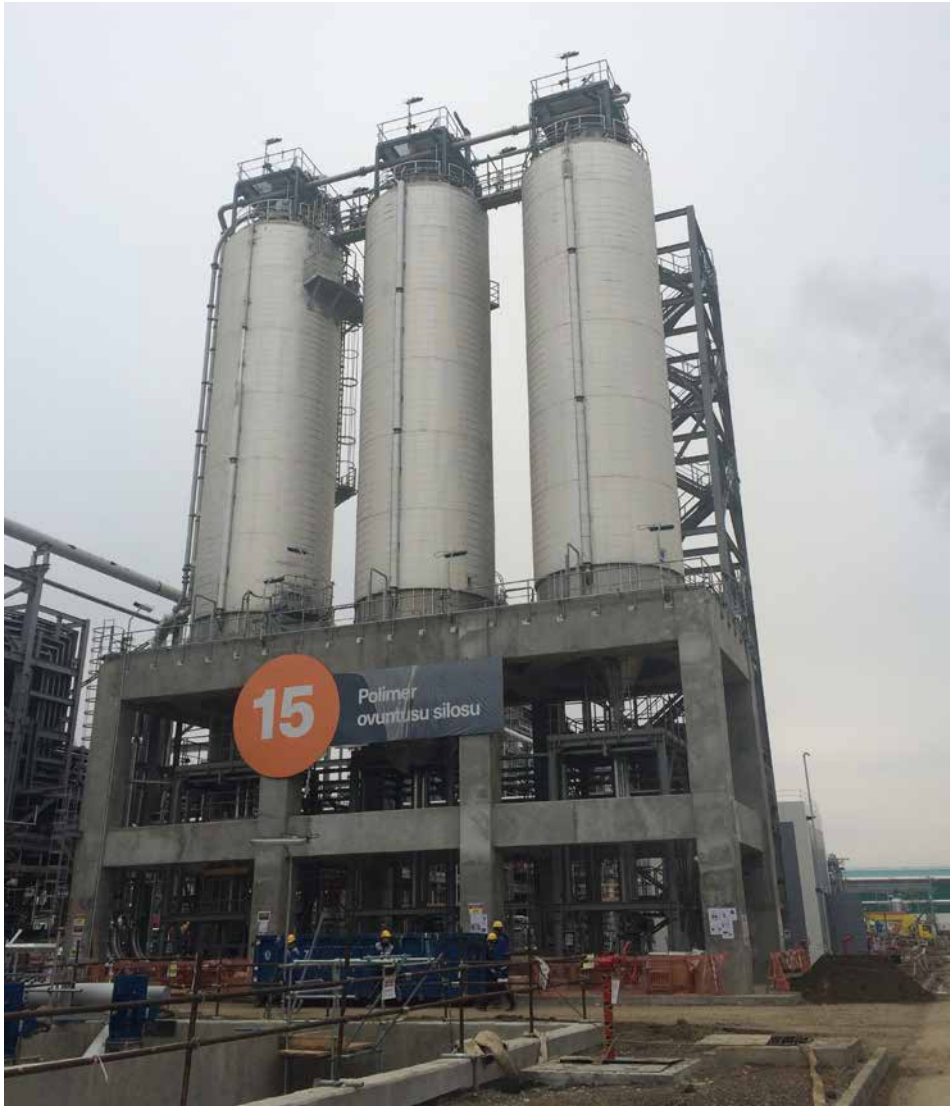
PP/U&O: PP Dry section / Powder Silos. Pre-commissioning activities in progress
