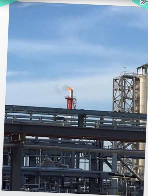
Flare Stack activated
