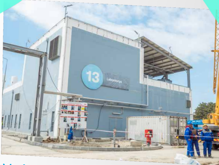
Mechanical completion of the laboratory
