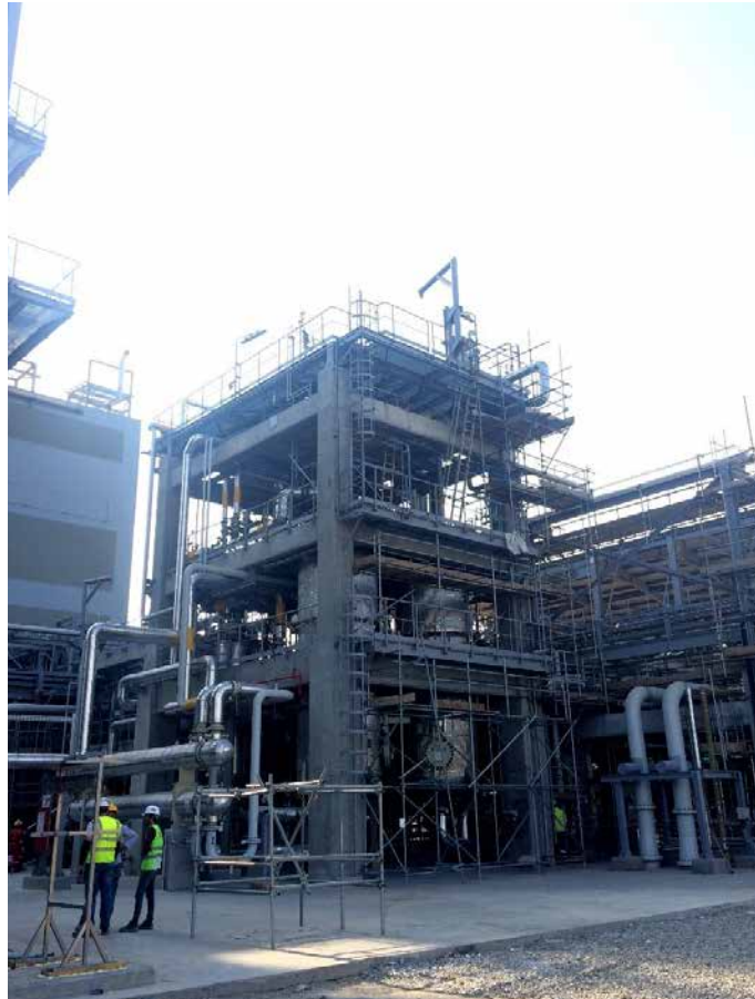
HDPE: Ethylene Treatment. Piping insulation and painting works ongoing
