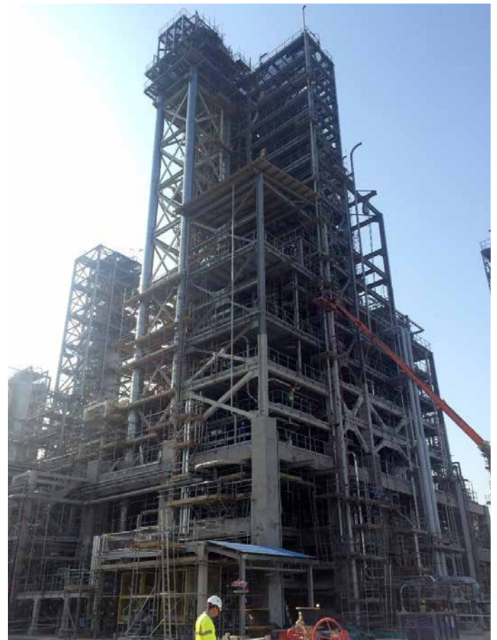
HDPE: Polymerization. Structural fire-proofing completed. Piping insulation ongoing
