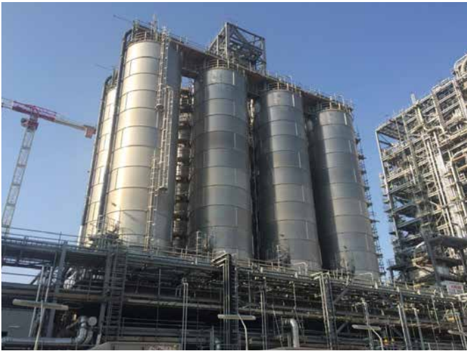
HDPE: Blending Silos. Piping insulation ongoing
