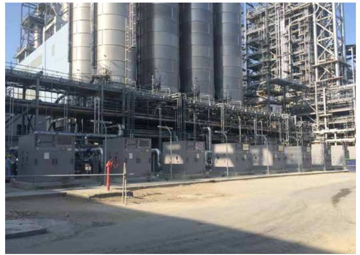
HDPE: Pellet blower package space for logistic conveying. Piping insulation ongoing
