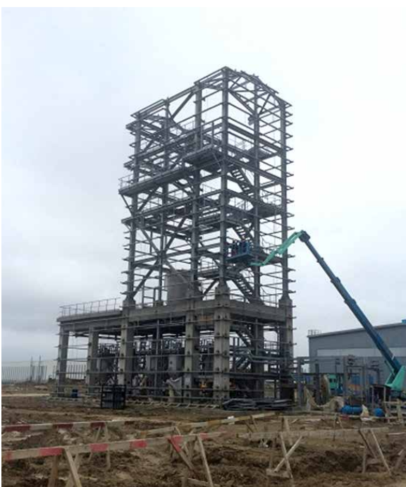
HDPE: Catalyst Activation. SS erection in progress
