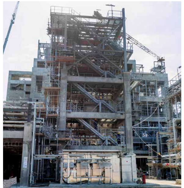
HDPE: Low Pressure Solvent Recovery. Instrument installation and cabling completed
