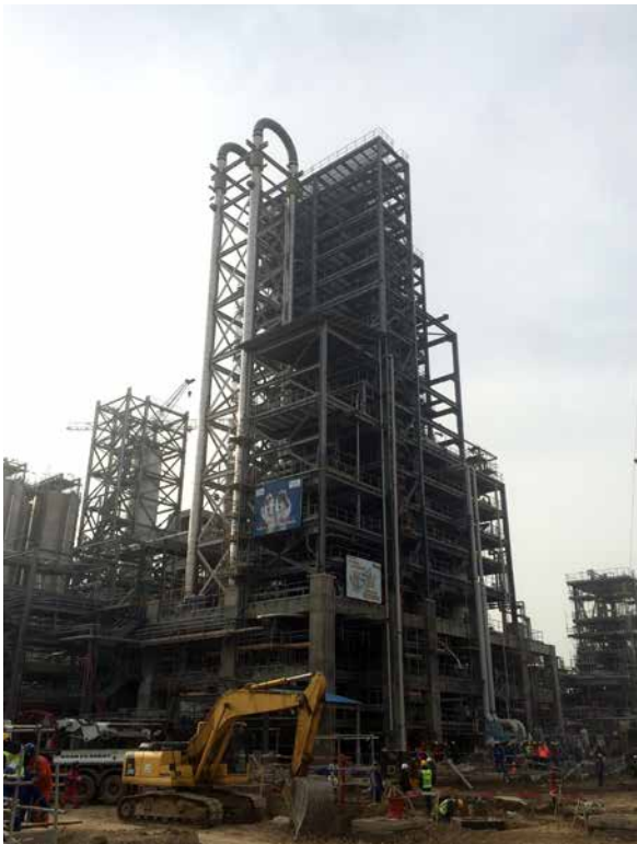
HDPE: Polymerization. Equipment erected. Piping & Support erection ongoing. SS, junction box, lighting, etc. installation in progress
