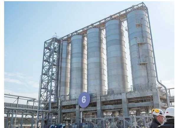
PP/U&O: Homogenization / Blender Silos. Commissioning activities in progress
