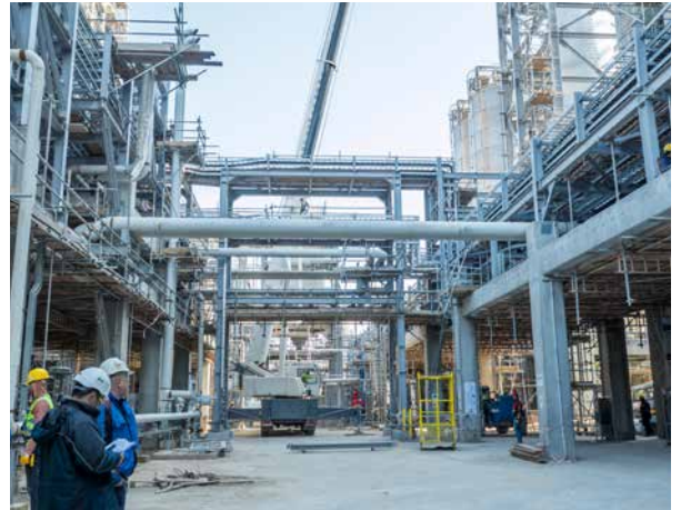
HDPE: Polymerization Pipe Rack. Pipe support installation ongoing. Cable tray installation ongoing. Cable pulling in progress
