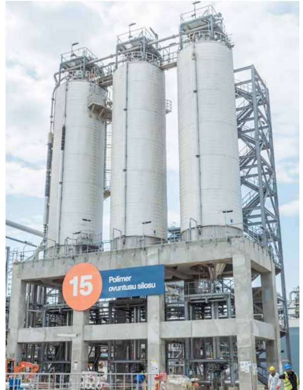
PP/U&O: PP Dry section / Powder Silos. Pre-commissioning activities in progress
