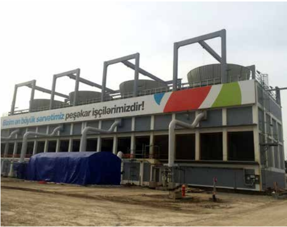
PP/U&O: Cooling Tower. Pre- commissioning activities in progress
