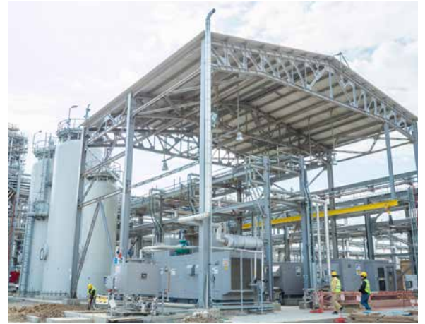
PP/U&O: Air/ HP Nitrogen Condensate Compressor Station's Storage & Pumping facilities. Pre- commissioning in progress
