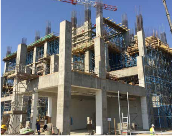
HDPE: Extrusion Structure. RCC works completed. Preparations for equipment installation started
