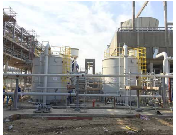
PP/U&O: Side Stream Filter Package. Pipe installation completed. Testing started
