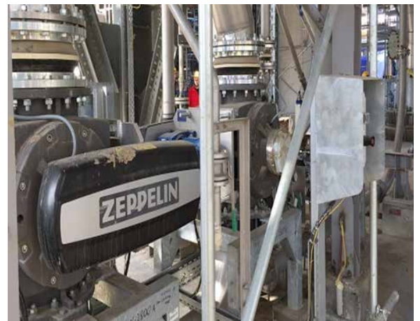
PP/U&O: PP- Wet section / Polymerization. Equipment installation and alignment ongoing. Installation of electrical instrumentation ongoing
