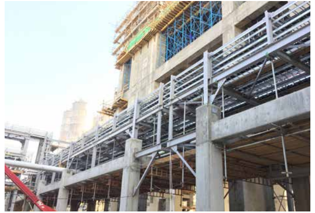
HDPE: Extrusion Pipe Rack. Pipe support installation ongoing. SS installation ongoing. Cable tray installation ongoing. Cable pulling started
