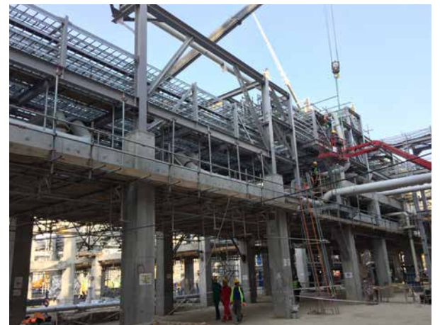
HDPE: Polymerization Pipe Rack. Pipe support installation ongoing. Cable tray installation ongoing. Cable pulling started
