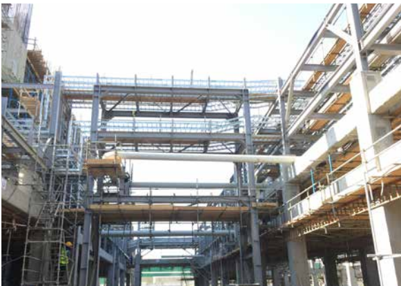
HDPE: Solvent recovery and Steam condensate area Piperack. Pipe support installation ongoing. Cable pulling started
