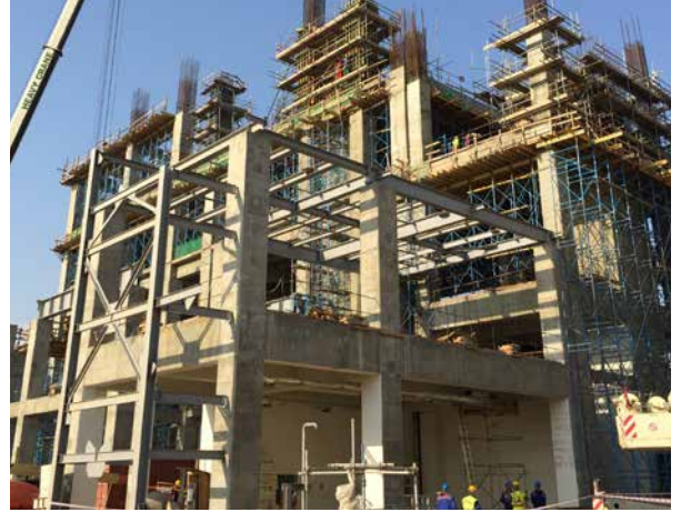
HDPE: Extrusion Structure. RCC works completed. Preparations for equipment installation started
