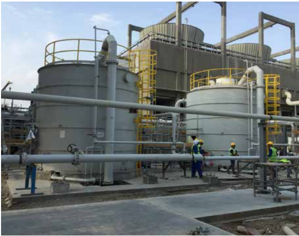
PP/U&O: Side Stream Filter Package. Pipe installation completed. Testing started
