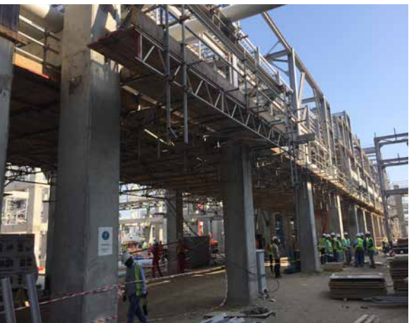
HDPE: Polymerization Pipe Rack. Pipe support installation ongoing. Cable tray installation ongoing. Cable pulling started
