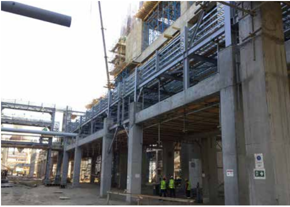
HDPE: Extrusion Pipe Rack. Pipe support installation ongoing. SS installation ongoing. Cable tray installation ongoing. Cable pulling started
