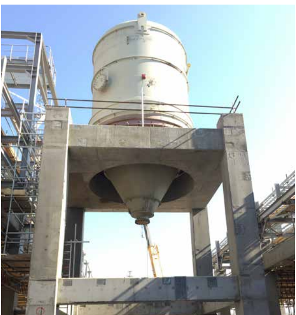
HDPE: Reactors Dump tank. Tank installation completed. Electrical and instrumentation works started
