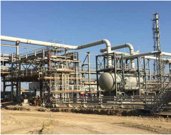
PP/U&O: Flare Knock Out Drum. Pipe testing ongoing. Equipment alignment ongoing. Electrical and instrumentation works started
