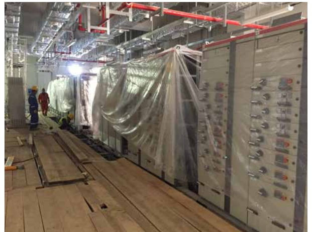
HDPE: Electrical Substation. Internal finishing and HVAC works ongoing. Electrical panel installation started
