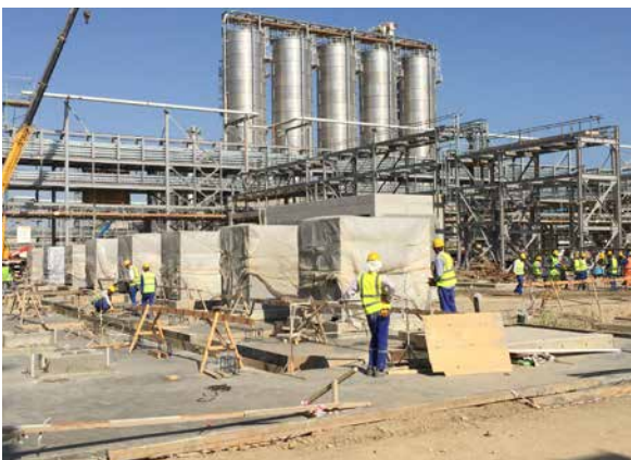
HDPE: Pellet blower package space for logistic conveying. Preparation works for equipment installation ongoing
