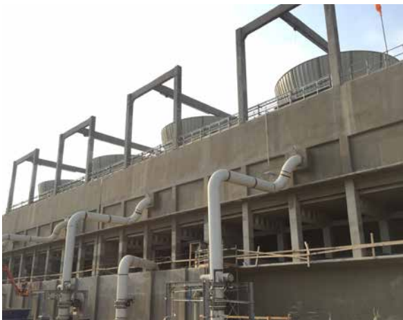
PP/U&O: Cooling Tower. Pipe and Equipment installation ongoing. Cable tray installation completed. Cable pulling and connecting ongoing. Façade painting started
