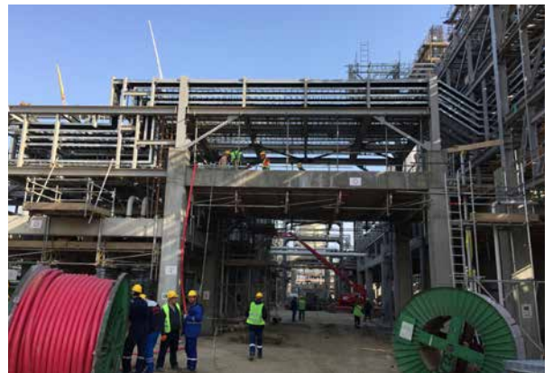
HDPE: Solvent recovery and Steam condensate area Piperack. Pipe support installation ongoing. Cable pulling started
