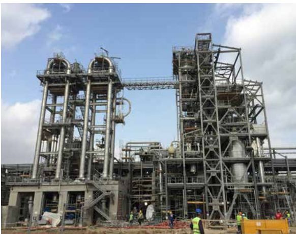
PP/U&O: PP- Wet section / Polymerization. Equipment installation and alignment ongoing. Installation of electrical instrumentation ongoing
