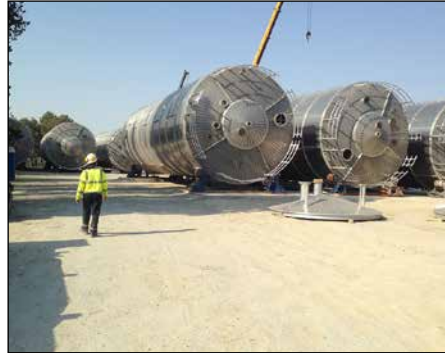
8 HDPE blending silos erected over a month p.18
