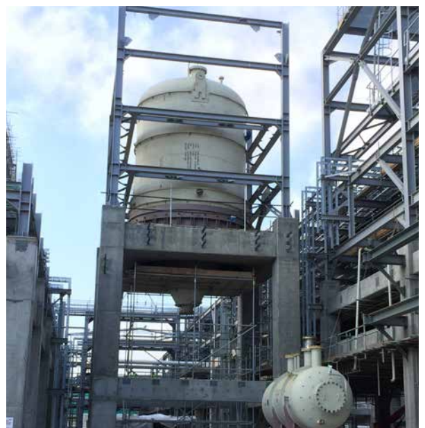
HDPE: Reactors Dump tank. Tank installation completed. Electrical and instrumentation works started
