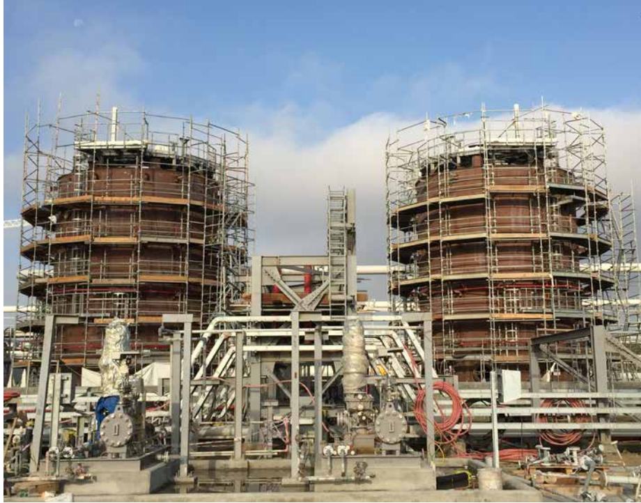
PP/U&O: Hexene Storage Tank. Tank erection ongoing. Piping works ongoing
