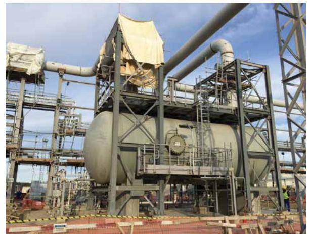
PP/U&O: Flare Knock Out Drum. Pipe testing, electrical and instrumentation works in progress
