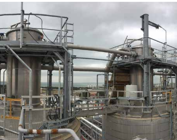
PP/U&O: PP Dry section / Powder Silos. Equipment and Pump alignment ongoing. Electrical and instrumentation works ongoing. Lighting installation in progress
