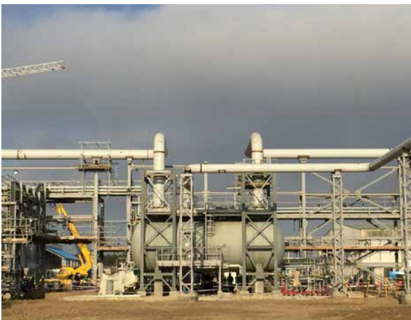
PP/U&O: Flare Knock Out Drum. Pipe testing, electrical and instrumentation works in progress
