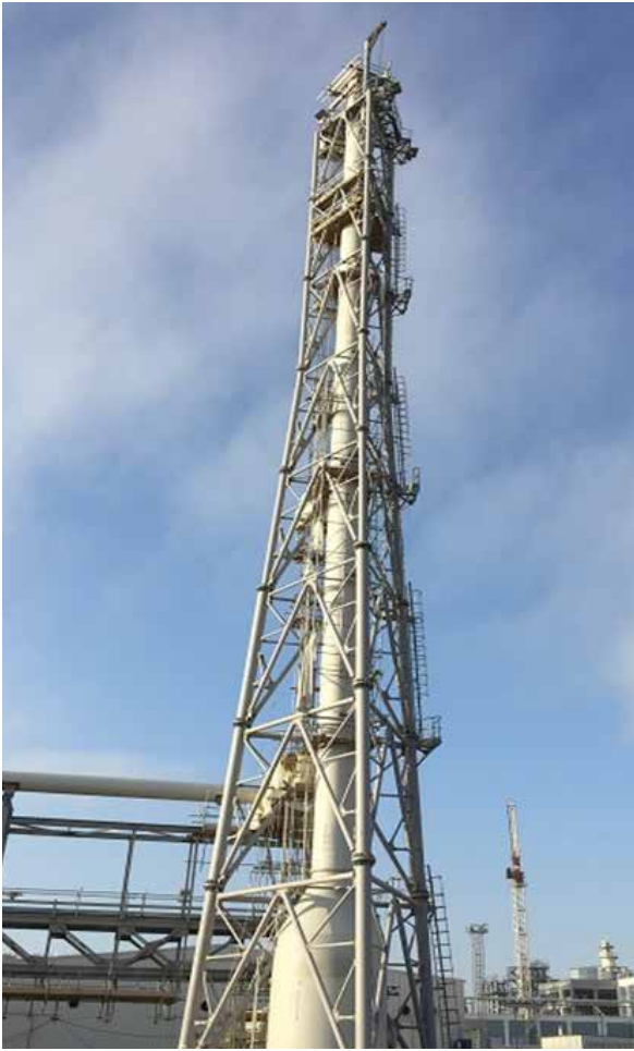
PP/U&O: Flare Stack. Commissioning completed
