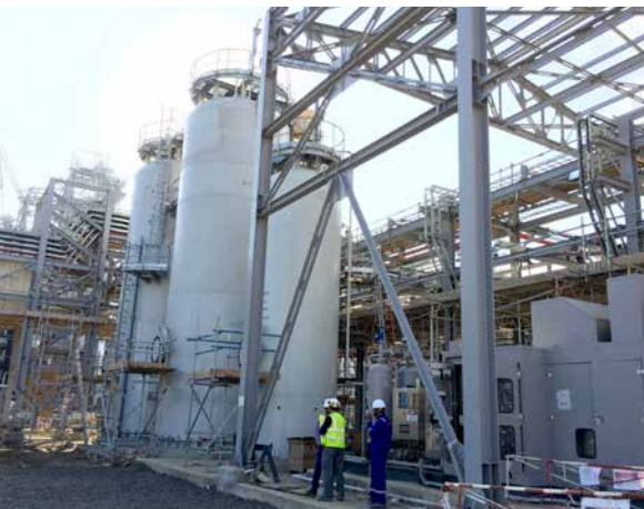
PP/U&O: Air/ HP Nitrogen Condensate Compressor Station Storage & Pumping. Equipment and pump alignment ongoing. Installation of electrical instrumentation ongoing
