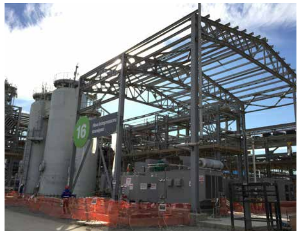
PP/U&O: Air/ HP Nitrogen Condensate Compressor Station Storage & Pumping. Equipment and pump alignment ongoing. Installation of electrical instrumentation ongoing
