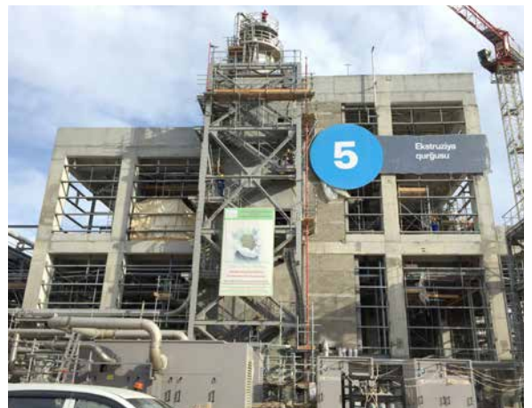
PP/U&O: PP Dry Section / Extrusion building. Equipment installation and alignment ongoing. Electrical and instrumentation works ongoing. Façade sheeting installation in progress
