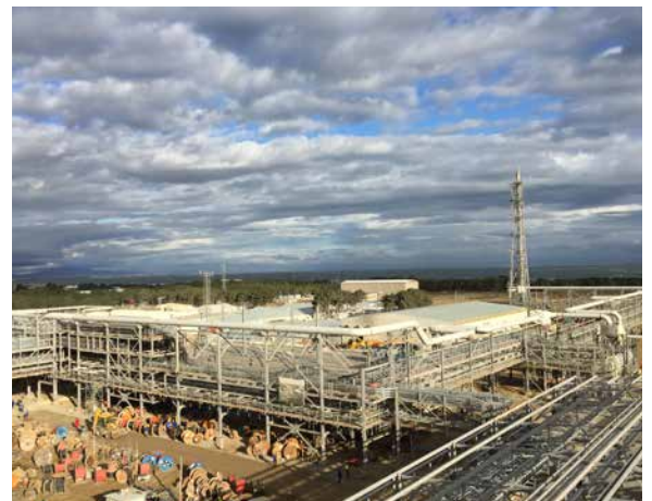
PP/U&O: Interconnecting Pipe Racks. Pipe erection ongoing. Cable pulling ongoing
