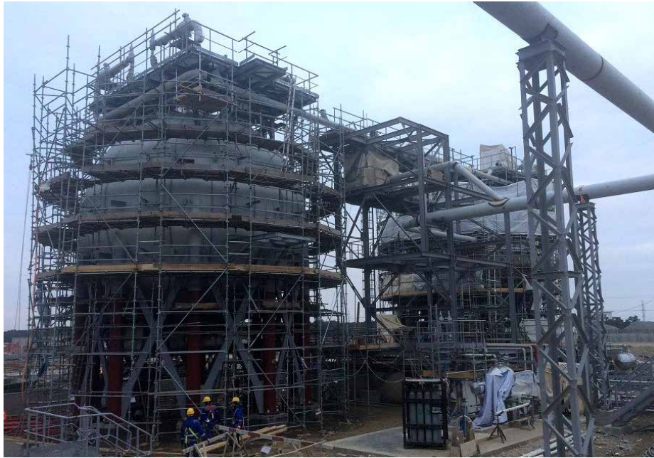
PP/U&O: Isobutane Sphere. Sprinkler system installation in progress
