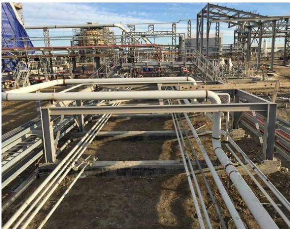
PP/U&O: Pipe Sleepers. Pipe erection and cable tray installation ongoing. Cable pulling ongoing
