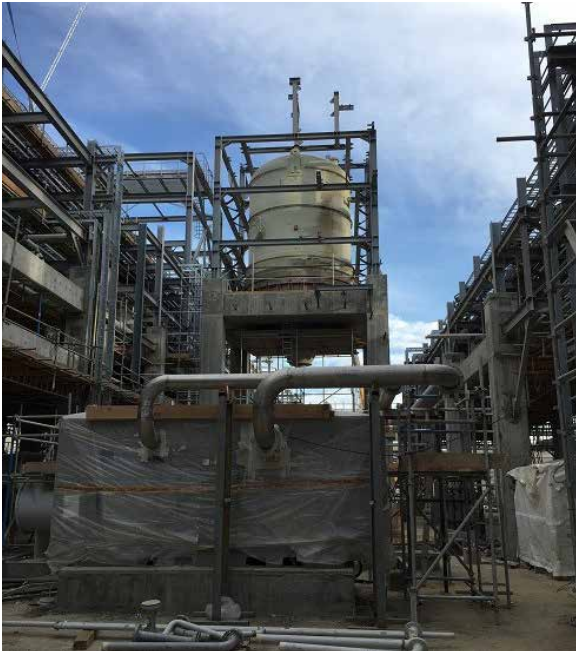
HDPE: Reactors Dump tank. Electrical and instrumentation works in progress
