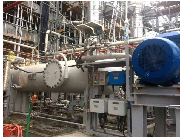
PP/U&O: PP-Wet section / Polymerization. Equipment installation and alignment ongoing. Installation of electrical instrumentation ongoing. Piping test in progress
