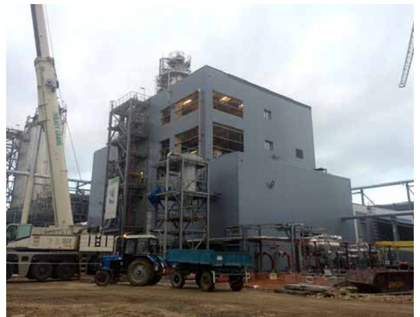
PP/U&O: PP Dry Section / Extrusion building. Equipment installation and alignment ongoing. Electrical and instrumentation works ongoing. Most cladding work completed. Lift erection in progress
