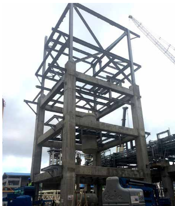
HDPE: Low Pressure Solvent Recovery. SS erection in progress. Paving completed
