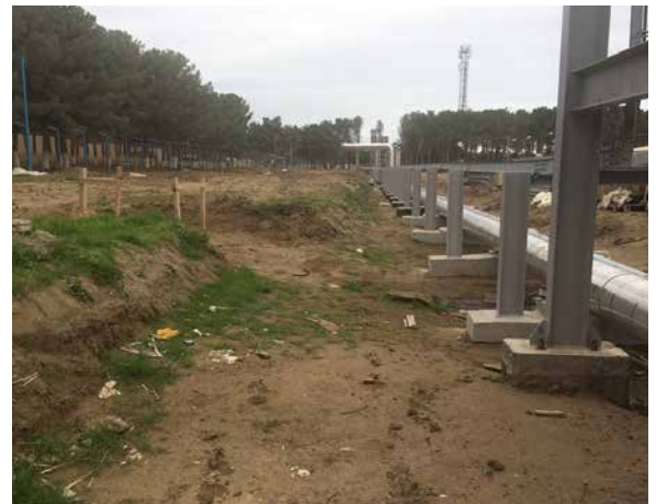
PP/U&O: Pipe Sleepers. Pipe erection and cable tray installation ongoing. Cable pulling ongoing
