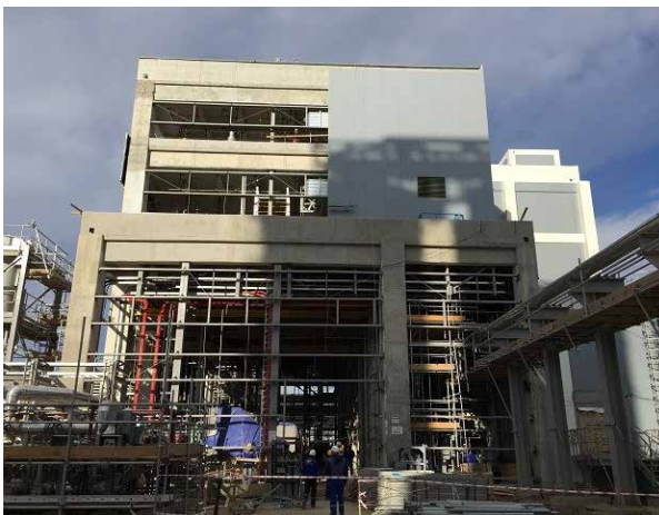
PP/U&O: PP Dry Section / Extrusion building. Equipment installation and alignment ongoing. Electrical and instrumentation works ongoing. Most cladding work completed. Lift erection in progress
