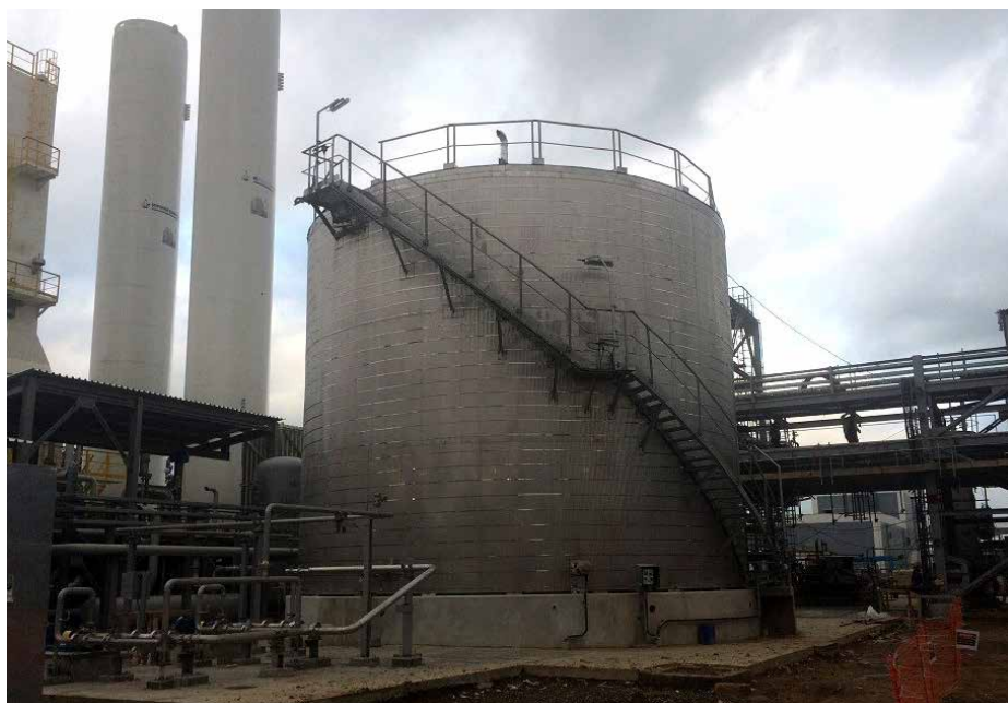
PP/U&O: DM Water Storage Tank. Pre-commissioning in progress
