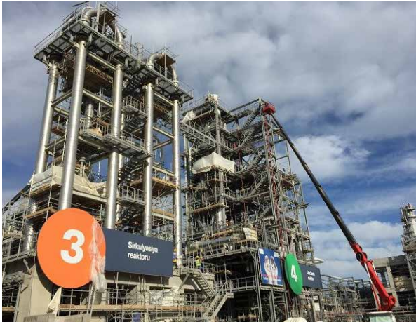
PP/U&O: PP-Wet section / Polymerization. Equipment installation and alignment ongoing. Installation of electrical instrumentation ongoing. Piping test in progress
