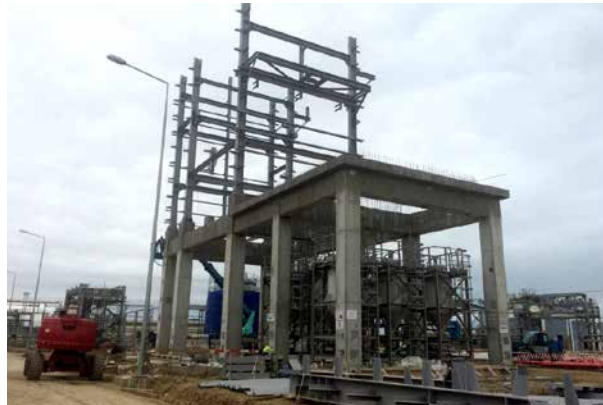
HDPE: Catalyst Activation. SS erection in progress
