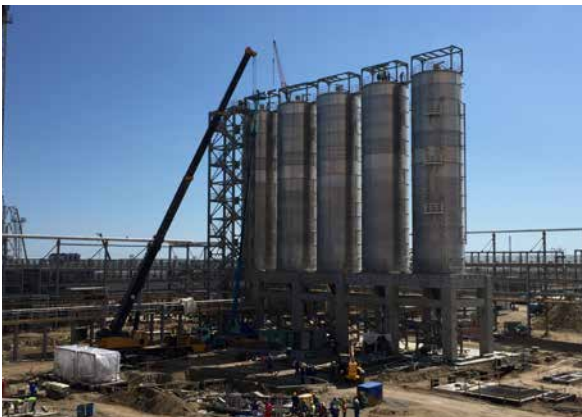
PP/U&O: Homogenization / Blender Silo. Pump, pipe and equipment installation started
