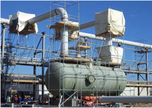
PP/U&O: Flare Knock Out Drum. Pipe connection ongoing
