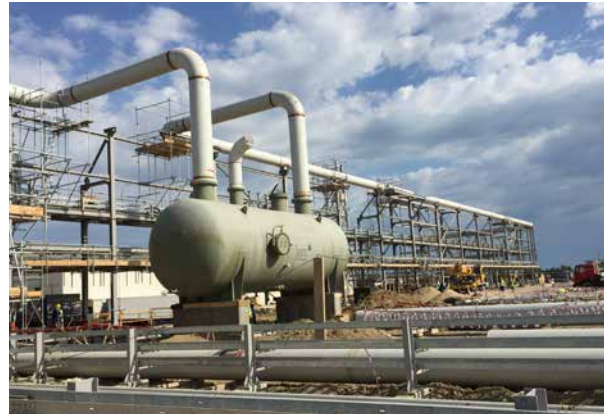
PP/U&O: Flare Knock Out Drum. Pipe connection ongoing
