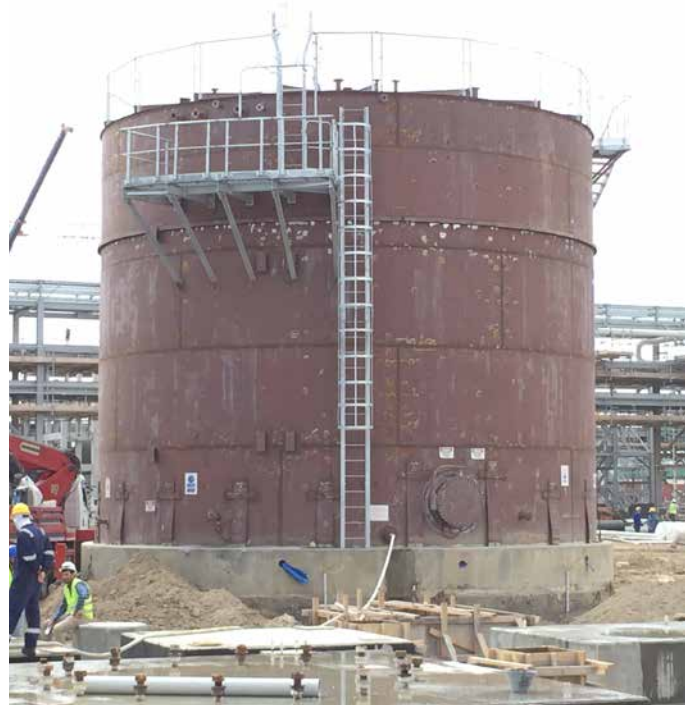
PP/U&O: DM Water Storage Tank. Leak test conducted
