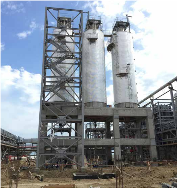
PP/U&O: PP Dry /Powder Silo. Equipment installation started
