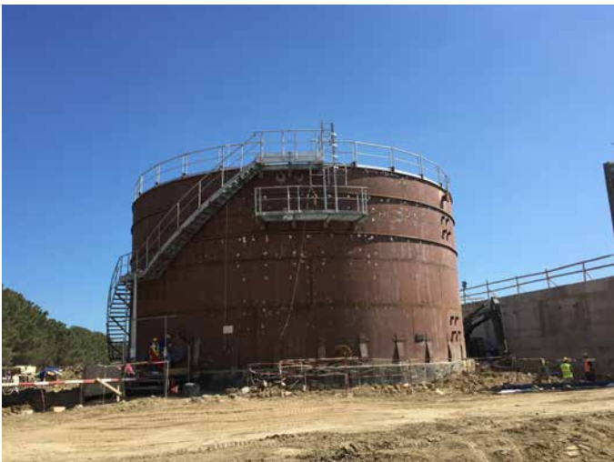
PP/U&O: Raw Water Storage Tank. Leak test conducted
