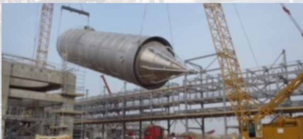
Blending Silos installation under way
