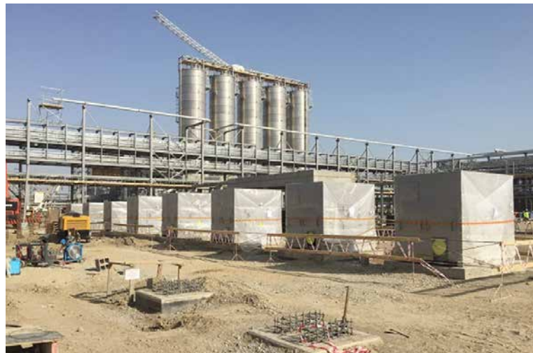
HDPE: Pellet blower package space for logistic conveying. Equipment was installed
