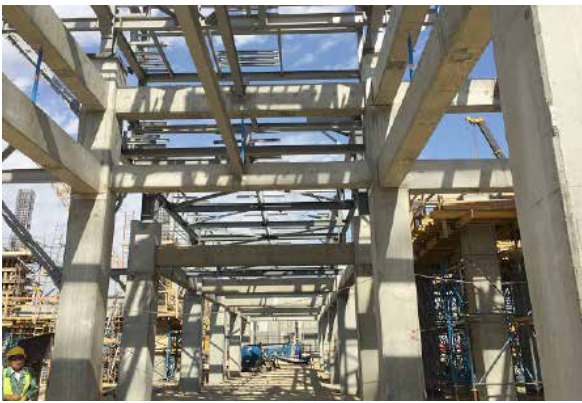
HDPE: Extrusion Pipe Rack. RCC works completed. Pipe support installation started
