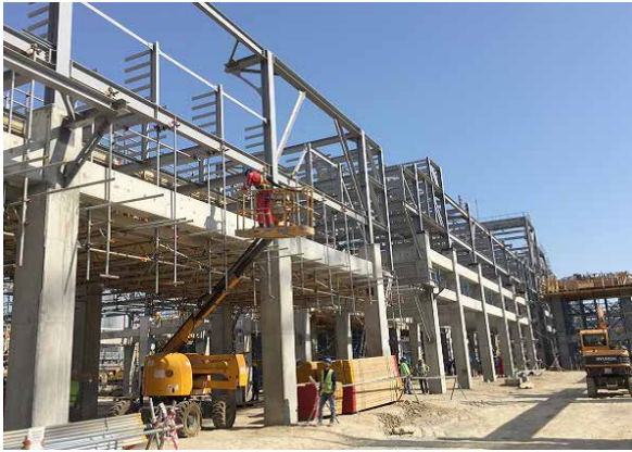
HDPE: Solvent recovery and Steam condensate area Piperack. Pipe support installing started
