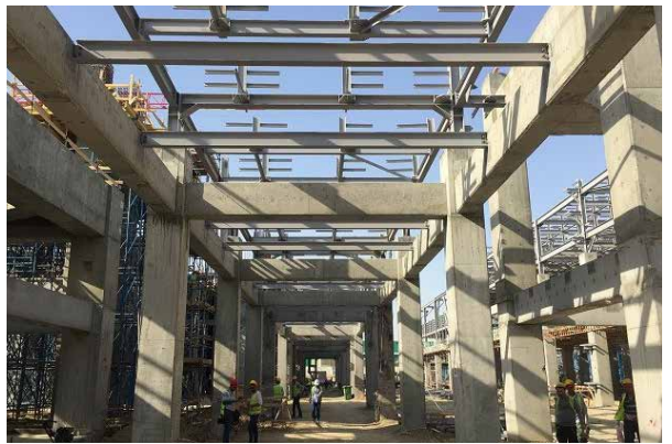
HDPE: Polymerization Pipe Rack. Pipe support installing started
