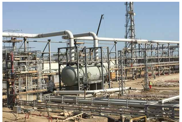
PP/U&O: Flare Knock Out Drum. Pump installed. Pipe connection ongoing
