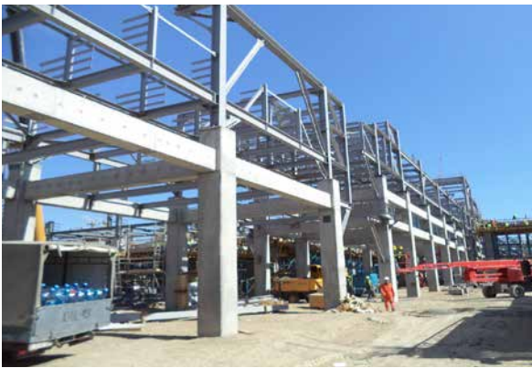
HDPE: Polymerization Pipe Rack. Pipe support installing started
