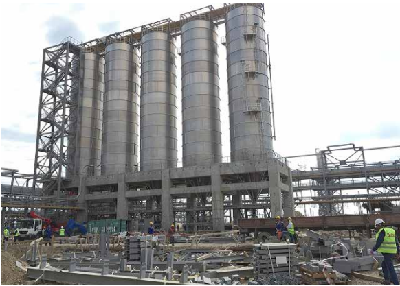
PP/U&O: Homogenization / Blender Silo. Pump, pipe and equipment alignment started
