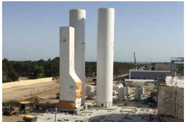
Nitrogen package. Tank installation completed. Started preparing foundation for equipment installation
