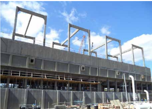
PP/U&O: Cooling Tower. Sprinkler installation ongoing. Pipe and equipment installation ongoing. Fan installation started
