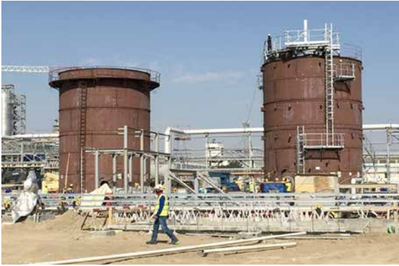
PP/U&O: Hexene Storage Tank. Tank erection ongoing
