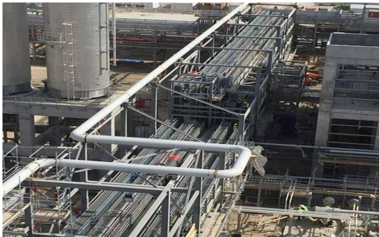
PP/U&O: Interconnecting Pipe Racks. Pipe erection ongoing. Cable pulling started
