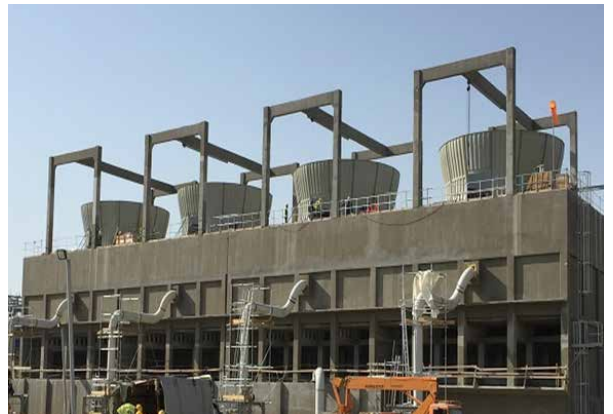
PP/U&O: Cooling Tower. Sprinkler installation ongoing. Pipe and equipment installation ongoing. Fan installation started
