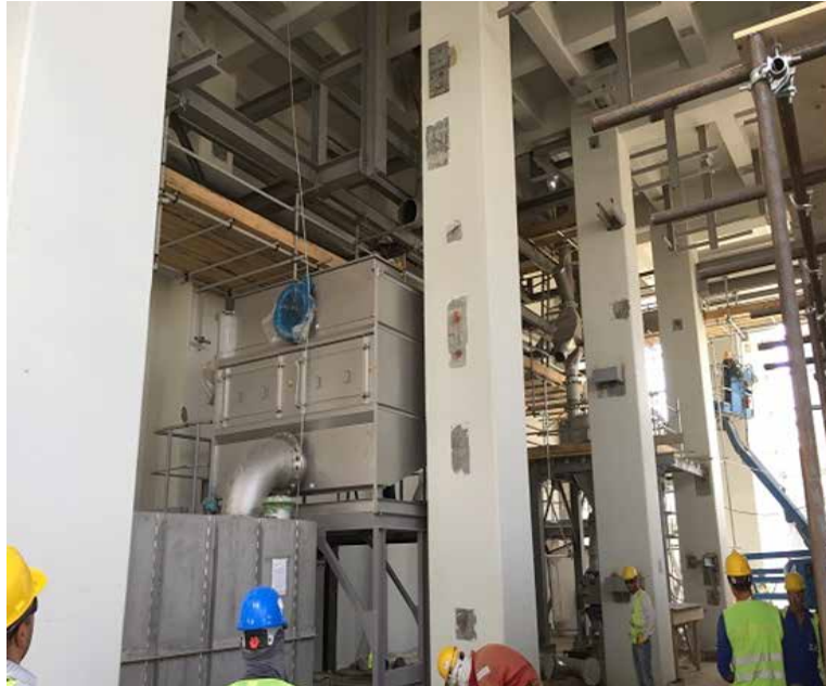
PP/U&O: Extrusion building. Equipment installation and alignment ongoing
