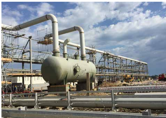
PP/U&O: Flare Knock Out Drum. Pump installed. Pipe connection ongoing
