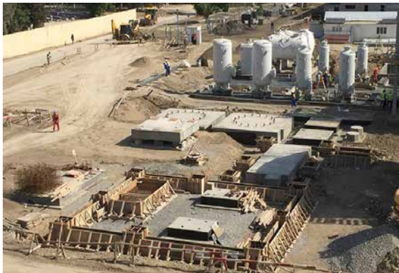
Nitrogen package. Tank installation completed. Started preparing foundation for equipment installation
