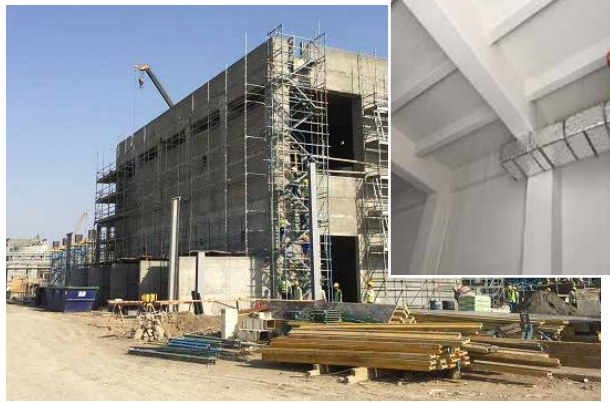
HDPE: Electrical Substation. RCC works completed. Finishing, Façade and HVAC works started
