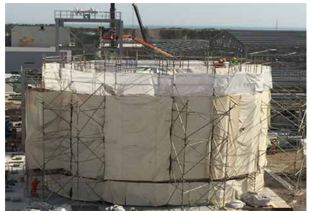
PP/U&O: DM Water Storage Tank. Tank painting started
