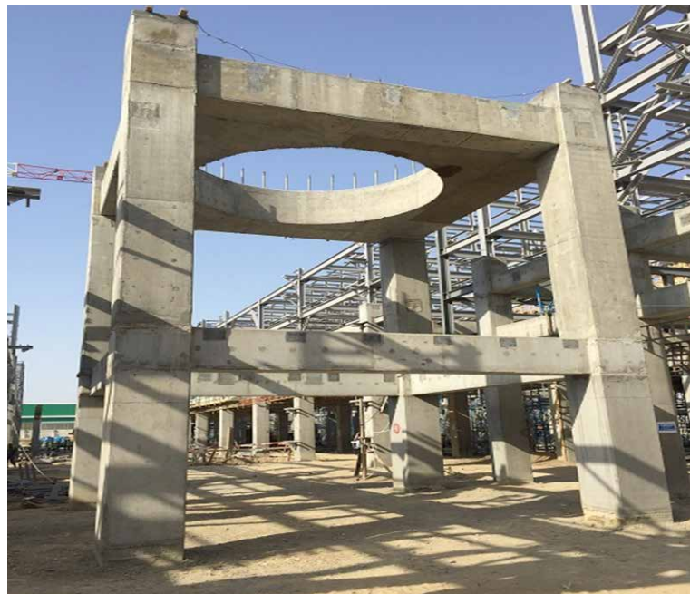
HDPE: Reactors Dump tank. Ready for tank installation
