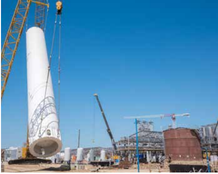
Delivery and installation of Nitrogen Storage Tank
