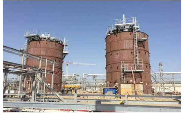
PP/U&O: Hexene Storage Tank. Tank erection ongoing
