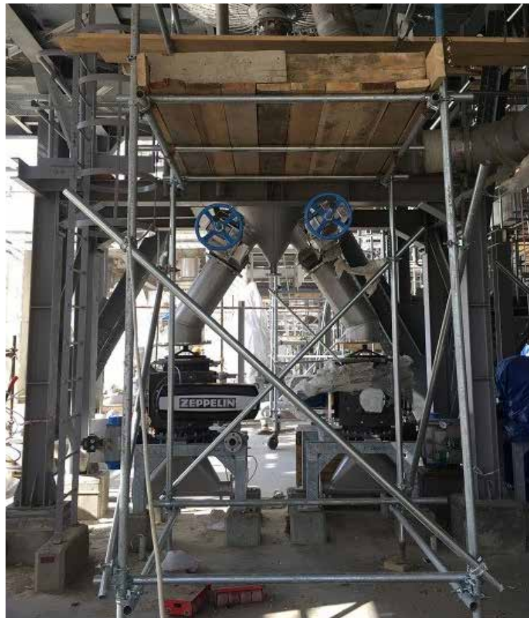
PP/U&O: PP-Wet section / Polymerization. Equipment installation and alignment ongoing
