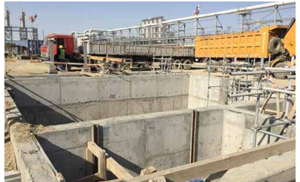
PP/U&O: Impounding Basin for Isobutane. Backfilling completed. Pump installation started
