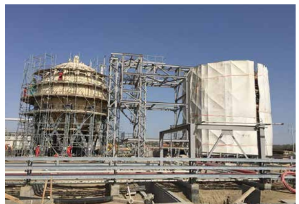
PP/U&O: Isobutane Sphere. Dike wall welding ongoing
