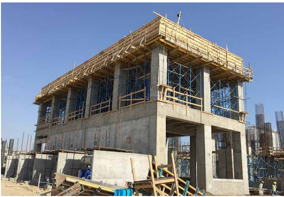
HDPE: Electrical Substation. RCC works completed. Finishing, Façade and HVAC works started
