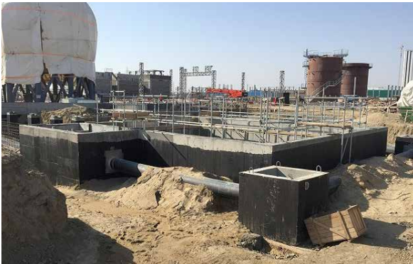
PP/U&O: Impounding Basin for Isobutane. Backfilling completed. Pump installation started
