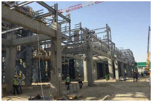
HDPE: Extrusion Pipe Rack. RCC works completed. Pipe support installation started
