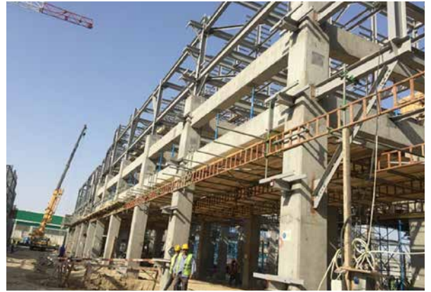
HDPE: Solvent recovery and Steam condensate area Piperack. Pipe support installing started
