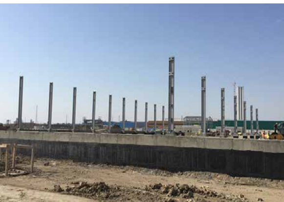
Warehouse. SS column installation ongoing. 102 columns installed. Backfilling ongoing. Heavy duty paving started. Valve house RCC work started
