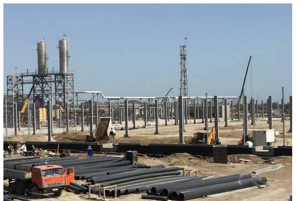
Warehouse. SS column installation ongoing. 102 columns installed. Backfilling ongoing. Heavy duty paving started. Valve house RCC work started
