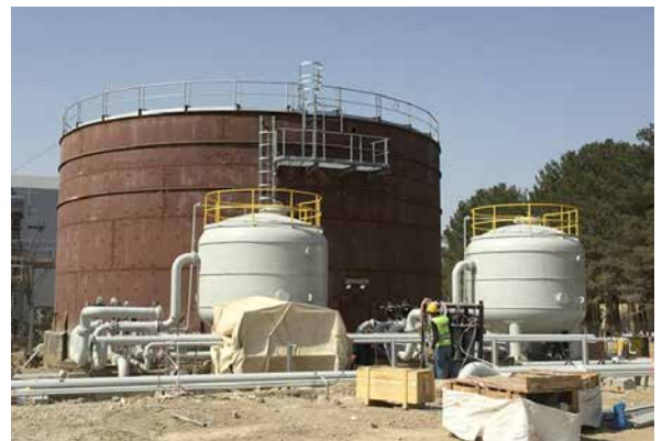
PP/U&O: Raw Water Storage Tank. Pipe installation started
