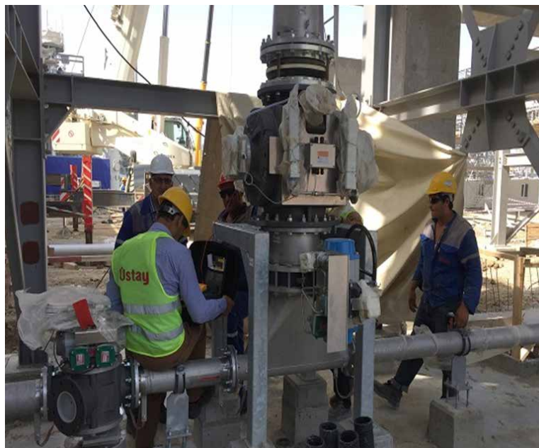
PP/U&O: PP Dry section / Powder Silo. Equipment and pump alignment started
