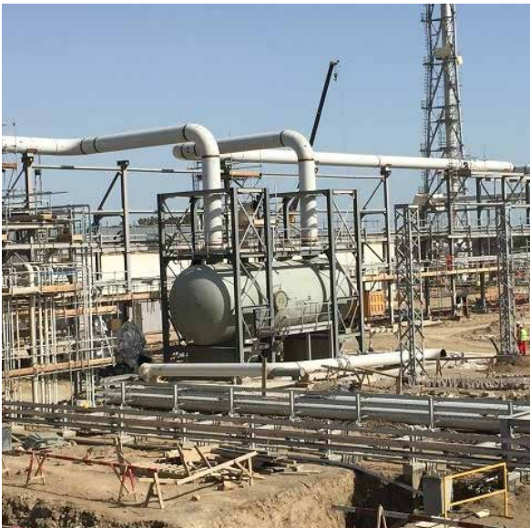
PP/U&O: Flare Knock Out Drum. Pipe connection ongoing
