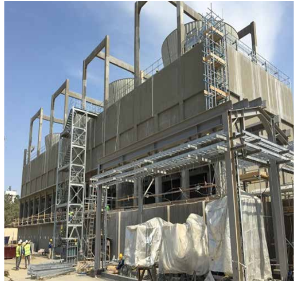
PP/U&O: Cooling Tower. Sprinkling system installation ongoing. Pipe and equipment installation ongoing. Fan installation completed. Cable tray installation started
