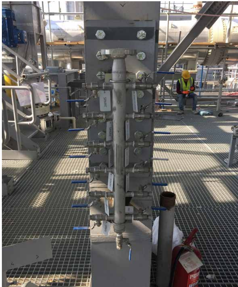
PP/U&O: PP Wet section / Polymerization. Equipment installation and alignment ongoing
