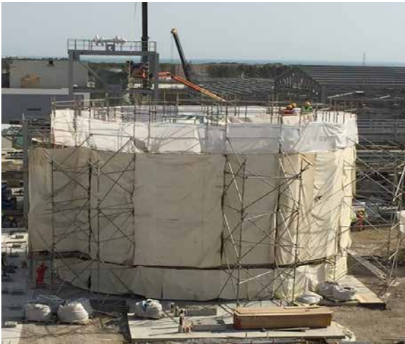
PP/U&O: DM Water Storage Tank. Tank painting ongoing
