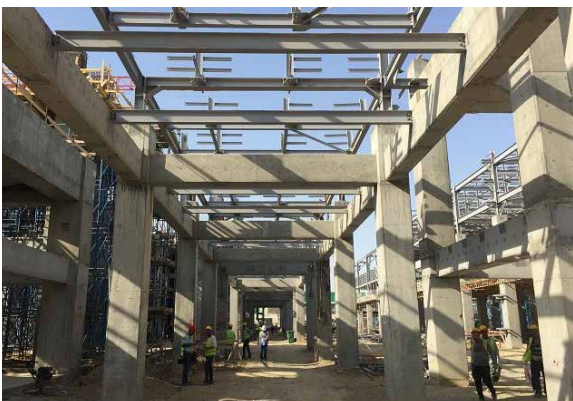
HDPE: Polymerization Pipe Rack. Pipe support installation ongoing
