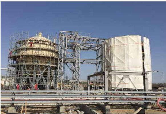
PP/U&O: Isobutane Sphere. Dike wall welding ongoing. Pipe installation started
