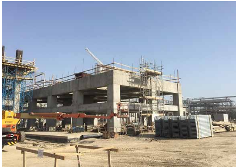
HDPE: Blending Silo. RCC works completed
