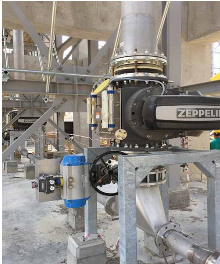
PP/U&O: PP Dry section / Powder Silo. Equipment and pump alignment ongoing
