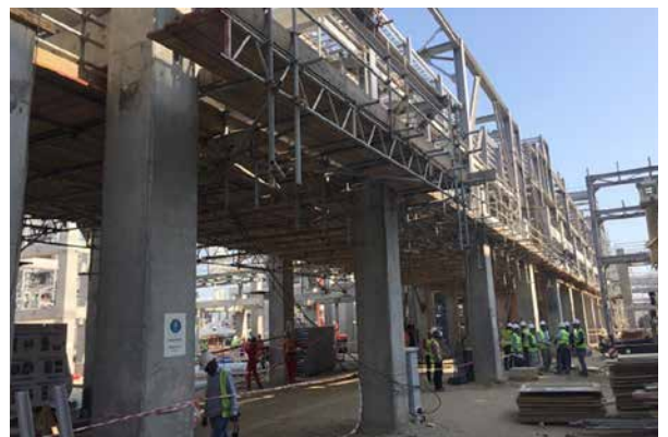
HDPE: Polymerization Pipe Rack. Pipe support installation ongoing
