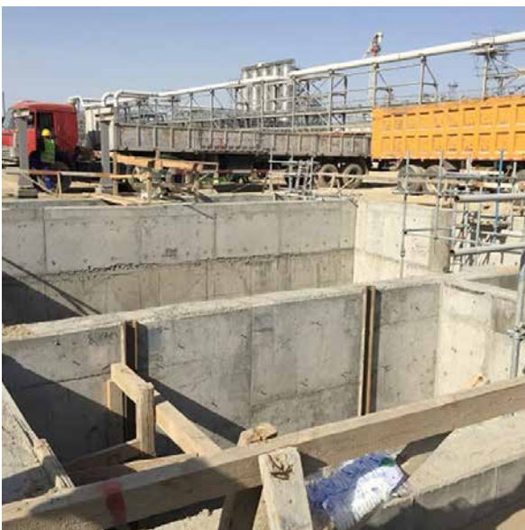
PP/U&O: Impounding Basin for Isobutane. Pump installation ongoing
