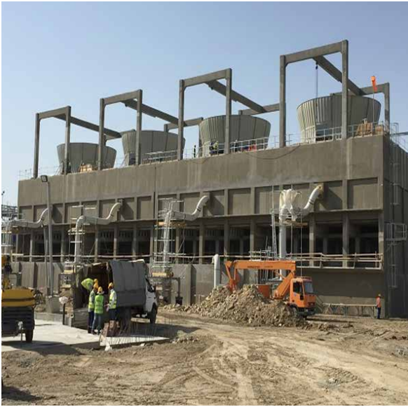
PP/U&O: Cooling Tower. Sprinkling system installation ongoing. Pipe and equipment installation ongoing. Fan installation completed. Cable tray installation started
