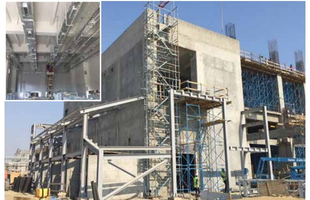
HDPE: Electrical Substation. Finishing, Façade and HVAC works ongoing
