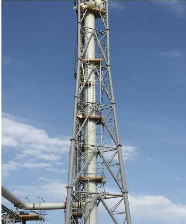
PP/U&O: Flare Stack. Equipment and derrick installation ongoing
