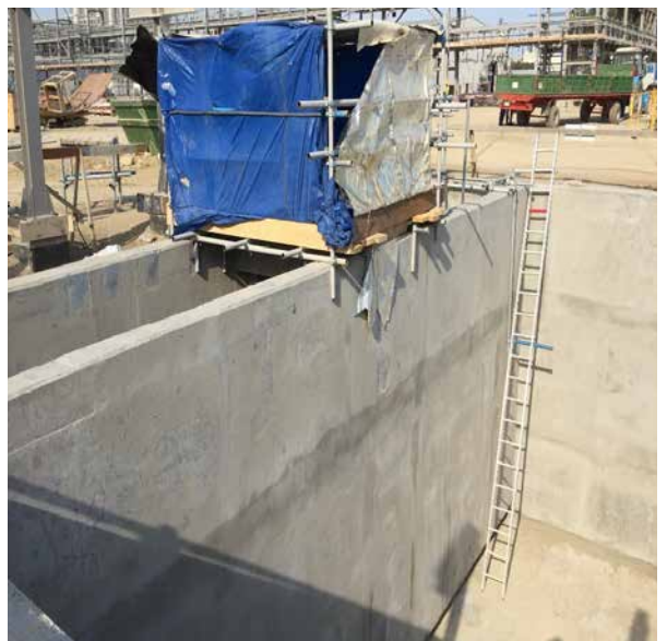
PP/U&O: Impounding Basin for Isobutane. Pump installation ongoing
