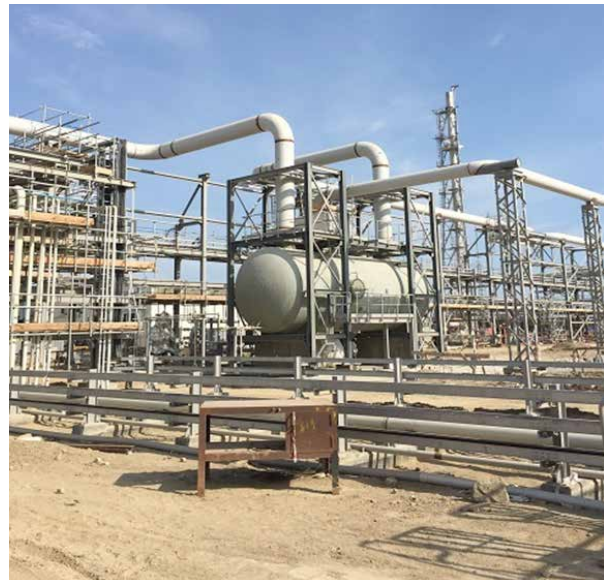
PP/U&O: Flare Knock Out Drum. Pipe connection ongoing
