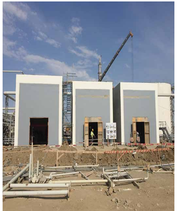
PP/U&O: Valve house. Valve and pipe installation ongoing. Façade painting started
