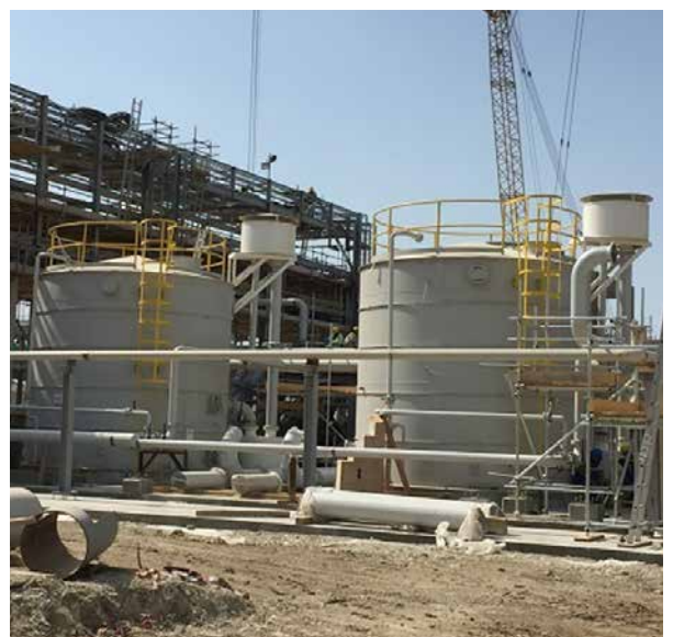
PP/U&O: Side Stream Filter Package. Pipe installation ongoing
