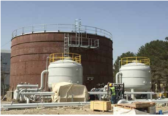
PP/U&O: Raw Water Storage Tank. Pipe installation ongoing
