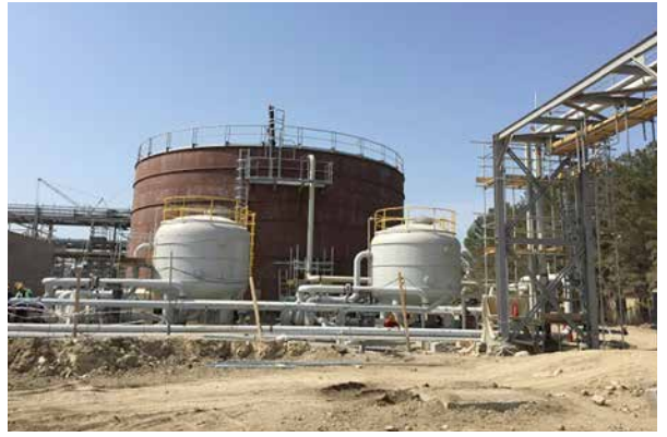
PP/U&O: Raw Water Storage Tank. Pipe installation ongoing
