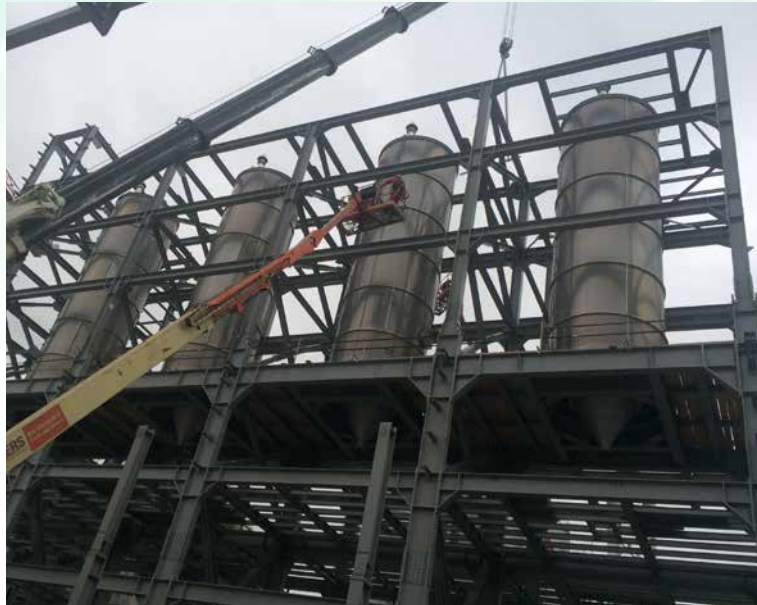
HDPE: Bagging & Packing. SS erection in progress
