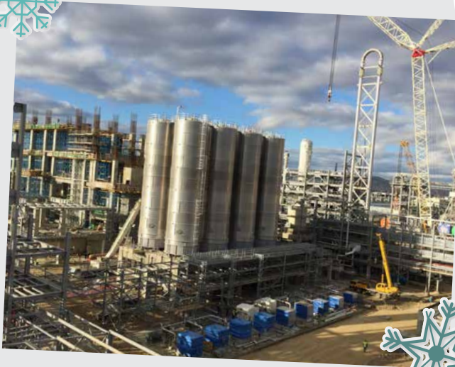
8 HDPE blending silos erected over a month
