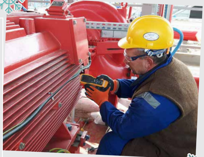
First Motor Solo Run activity performed
