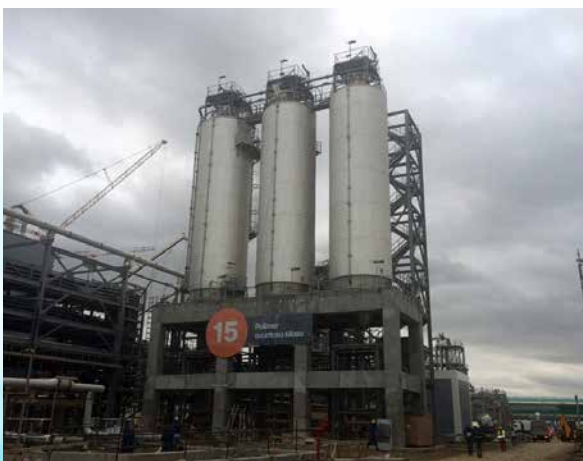
PP/U&O: PP Dry section / Powder Silos. Pre- commissioning activities in progress
