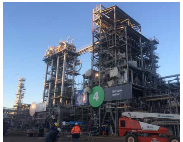
PP/U&O: PP- Wet section / Polymerization. Equipment testing in progress. Installation of electrical instrumentation ongoing. Piping test in progress. Branch cable tray installation in progress
