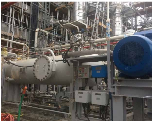
PP/U&O: PP- Wet section / Polymerization. Equipment testing in progress. Installation of electrical instrumentation ongoing. Piping test in progress. Branch cable tray installation in progress
