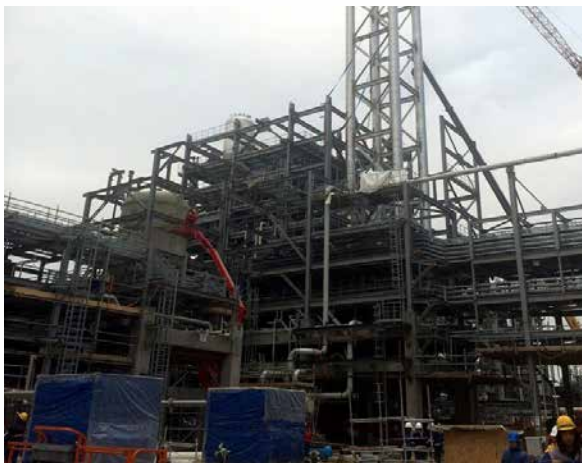
HDPE: Polymerization. Loop Reactor and Degasser installation completed. SS installation ongoing. Cable tray installation, piping and other works ongoing
