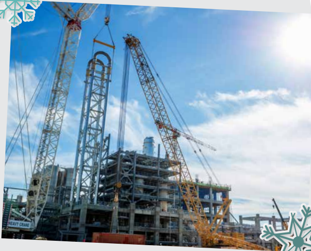
Installation of Loop Reactors
