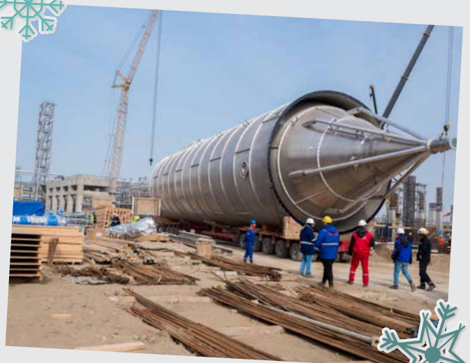
Blending Silos Installation
