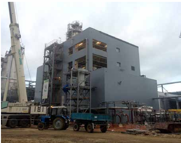
PP/U&O: PP Dry Section / Extrusion building. Suction system package installation in progress. Most cladding work completed. Lift erection in progress
