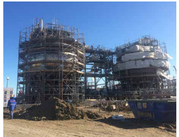
PP/U&O: Isobutane Sphere. Sprinkler system installation in progress
