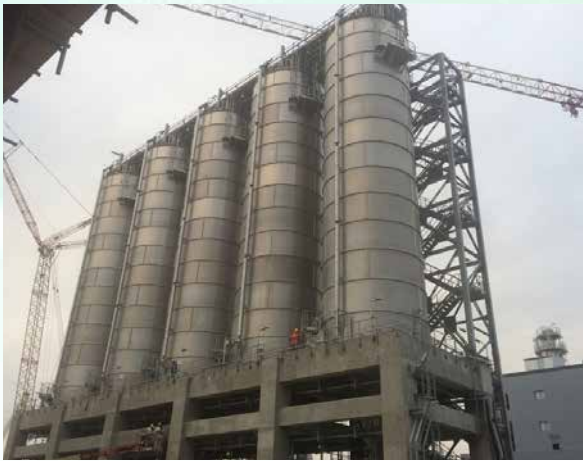
PP/U&O: Homogenization / Blender Silos. Pre- commissioning activities in progress
