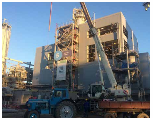
PP/U&O: PP Dry Section / Extrusion building. Suction system package installation in progress. Most cladding work completed. Lift erection in progress
