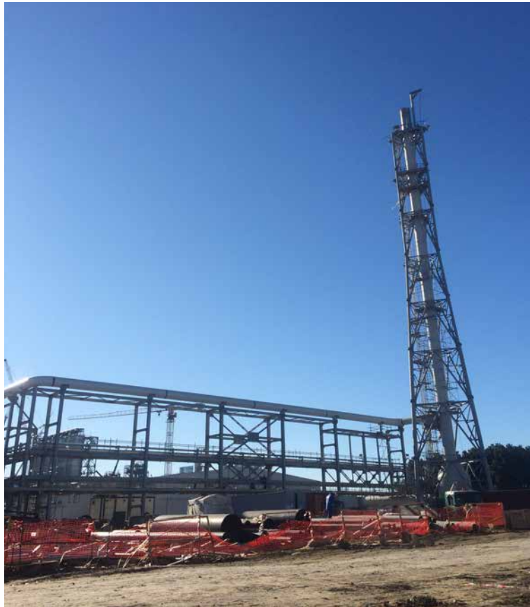
PP/U&O: Flare Stack. Pre-commissioning activities in progress
