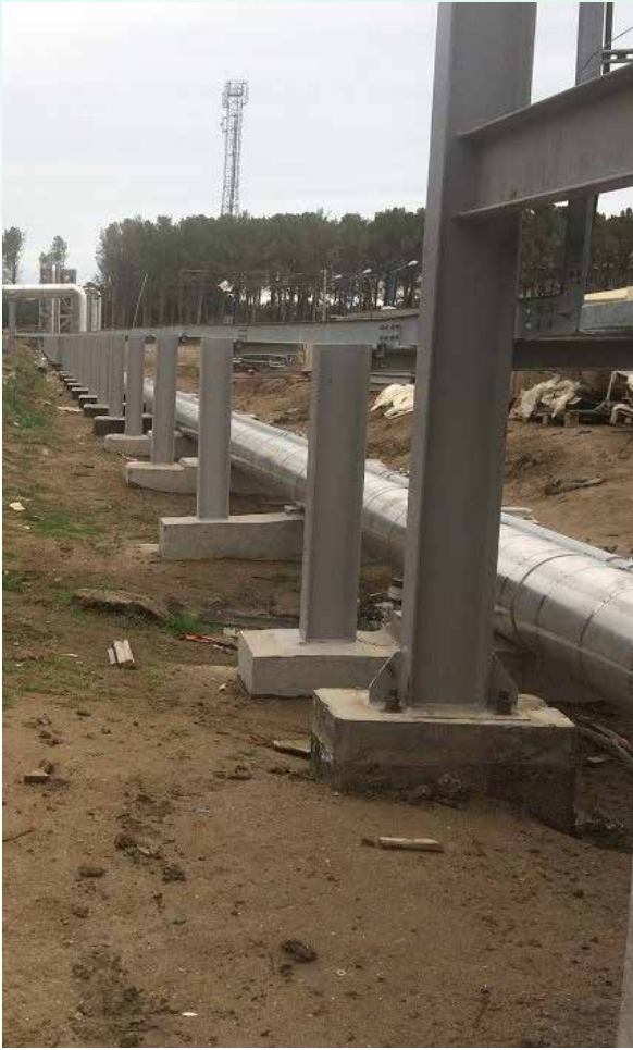
PP/U&O: Pipe Sleepers. Pipe erection and cable tray installation ongoing. Cable pulling ongoing
