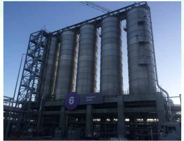
PP/U&O: Homogenization / Blender Silos. Pre- commissioning activities in progress
