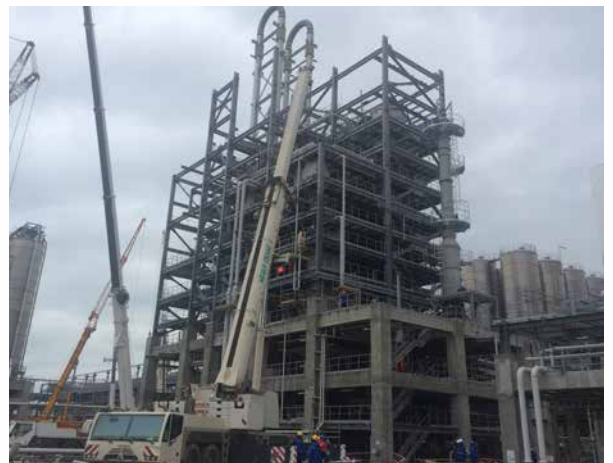
HDPE: Polymerization. Loop Reactor and Degasser installation completed. SS installation ongoing. Cable tray installation, piping and other works ongoing
