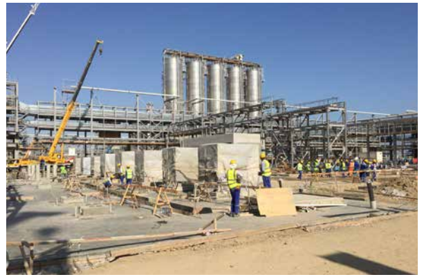
HDPE: Pellet blower package space for logistic conveying. Preparation works for equipment installation started
