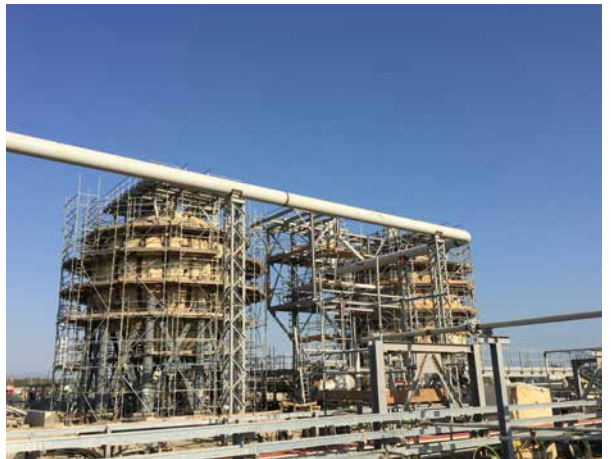
PP/U&O: Isobutane Sphere. Dike wall welding ongoing. Pipe installation ongoing
