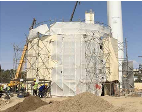
PP/U&O: DM Water Storage Tank. Tank painting completed. Thermal insulation works completed
