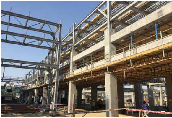
HDPE: Solvent recovery and Steam condensate area Piperack. Pipe support installation ongoing
