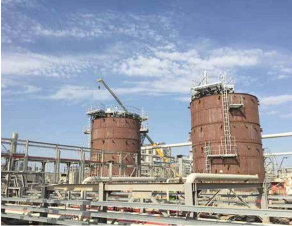
PP/U&O: Hexene Storage Tank. Tank erection ongoing. Piping works started
