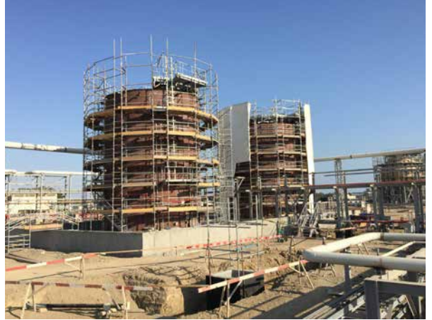
PP/U&O: Hexene Storage Tank. Tank erection ongoing. Piping works started
