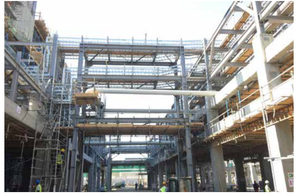
HDPE: Solvent recovery and Steam condensate area Piperack. Pipe support installation ongoing
