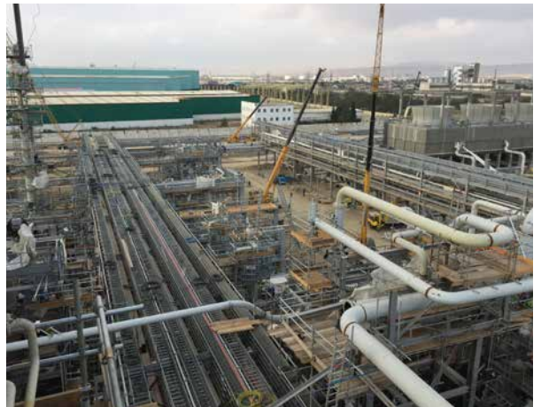
PP/U&O: Interconnecting Pipe Racks. Pipe erection ongoing. Cable pulling ongoing
