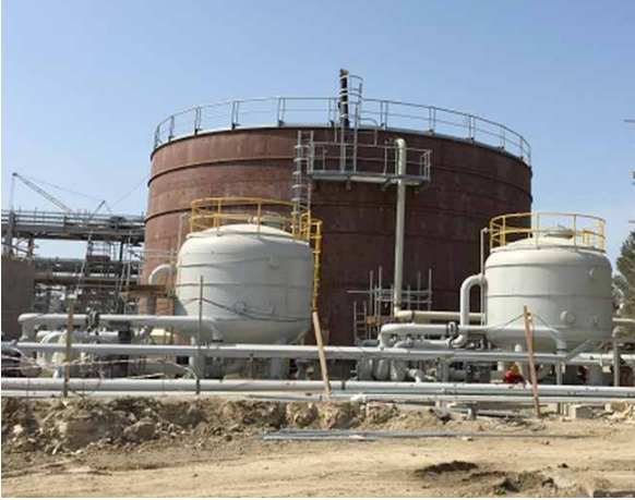
PP/U&O: Raw Water Storage Tank. Pipe installation ongoing
