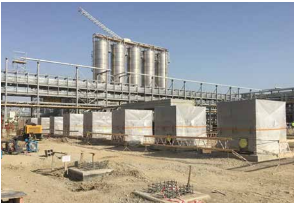
HDPE: Pellet blower package space for logistic conveying. Preparation works for equipment installation started
