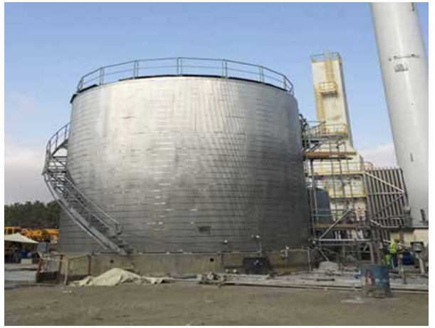
PP/U&O: DM Water Storage Tank. Tank painting completed. Thermal insulation works completed
