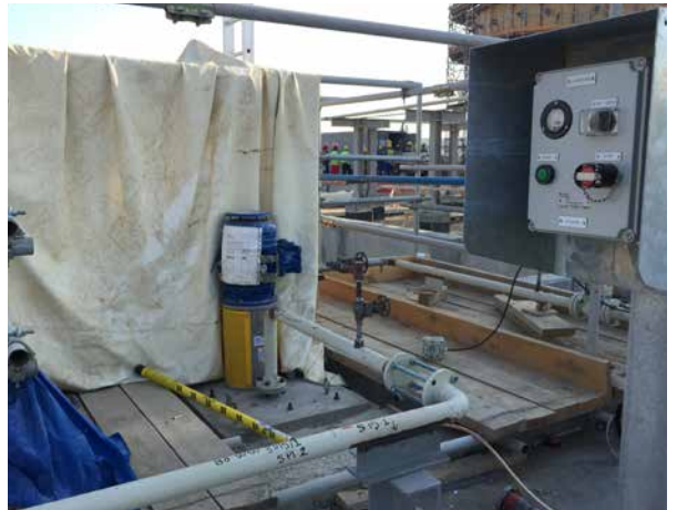
PP/U&O: Impounding Basin for Isobutane. Pump installation completed. Piping works started
