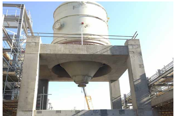
HDPE: Reactors Dump tank. Tank installation completed
