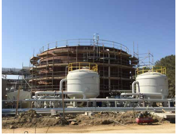
PP/U&O: Raw Water Storage Tank. Pipe installation ongoing
