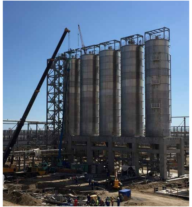
Homogenization / Blender Silo. Tank installation completed
