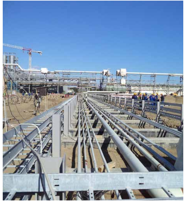
Pipe Sleepers. Piping and cable tray installation ongoing
