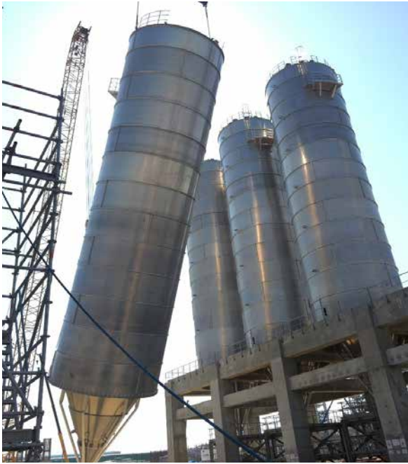
Homogenization / Blender Silo. Tank installation completed
