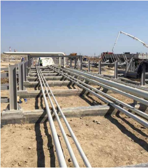
Pipe Sleepers. Piping and cable tray installation ongoing
