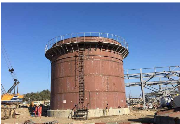
DM (demineralized) Water Storage Tank. Tank installation completed
