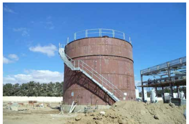
DM (demineralized) Water Storage Tank. Tank installation completed
