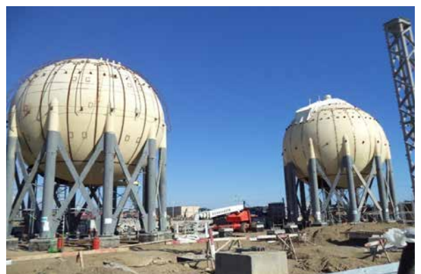
Isobutane Sphere. Pipe racks' installation started/ongoing
