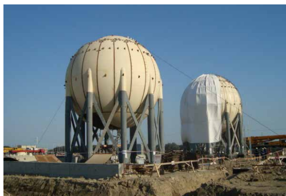
Isobutane Sphere. Pipe racks' installation started/ongoing
