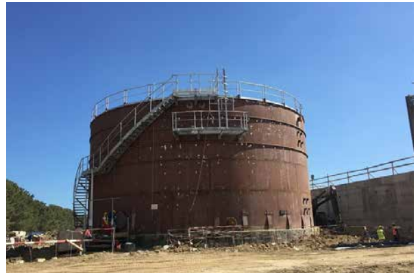
Raw Water Storage Tank. Tank installation completed
